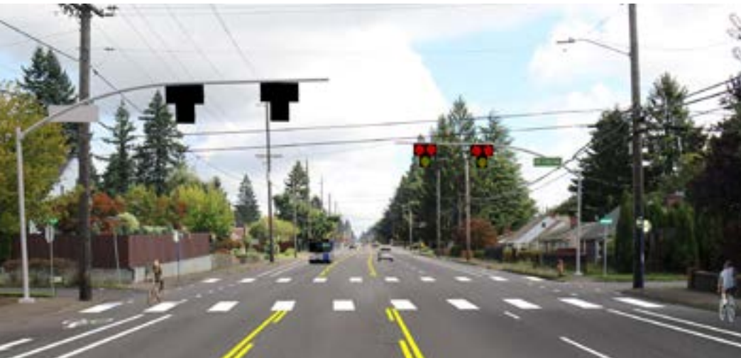
Proposed road reorg and new pedestrian hybrid signal at NE Glisan Street and 113th Avenue looking east. For more information visit: www.portland.gov/ .
