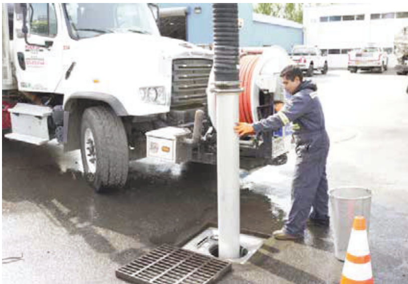
Catchbasin Cleaning Operation
