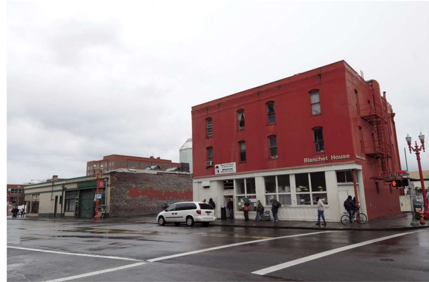
Old Blanchet House, in New Chinatown/Japantown, slated for demolition
