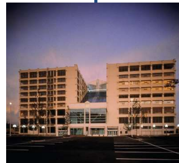
MONTGOMERY PARK ADAPTIVE REUSE
