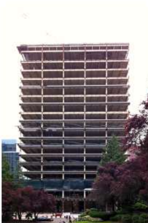
Demolition Complete - June 2011
