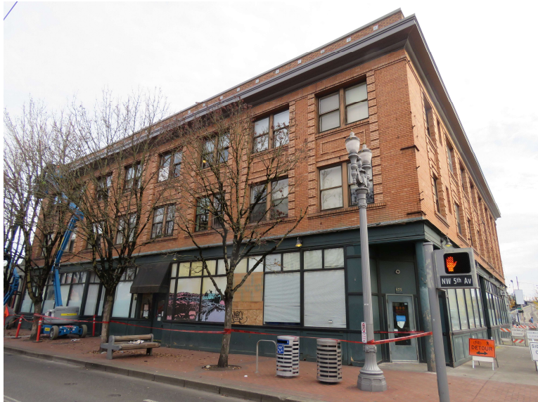
Central City Concern's Medford Hotel - 81 single occupancy units
