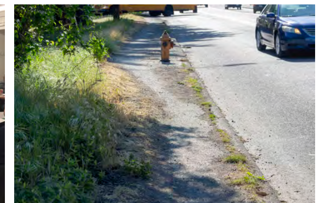
A photo of a deficient sidewalk in the corridor captured during a May 2019 field visit
