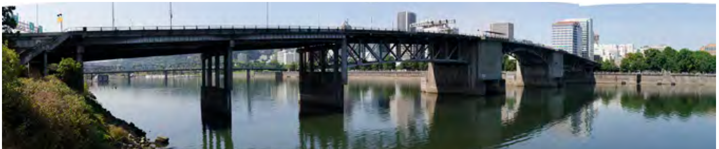
View from Eastbank Esplanade north of Morrison Bridge at SE Alder Street
