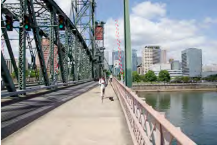
Viewpoint on Hawthorne Bridge north side center
