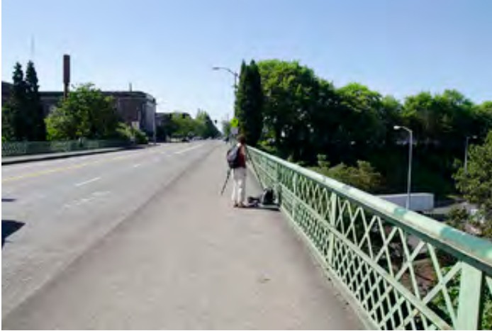
Viewpoint at NE 12th Avenue I-84 overpass
