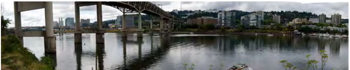
View from Greenway Trail (east) north of Marquam Bridge
