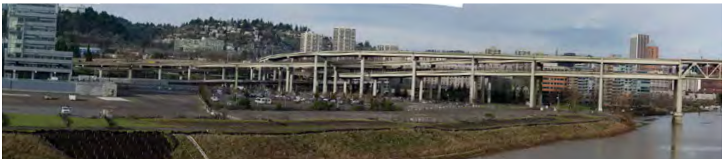
View from Tilikum Crossing, north side, west bump-out
