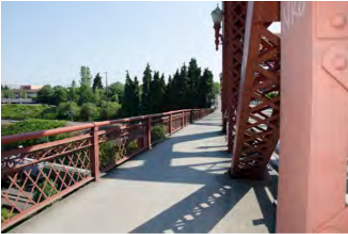
Viewpoint on Broadway Bridge north side east of center
