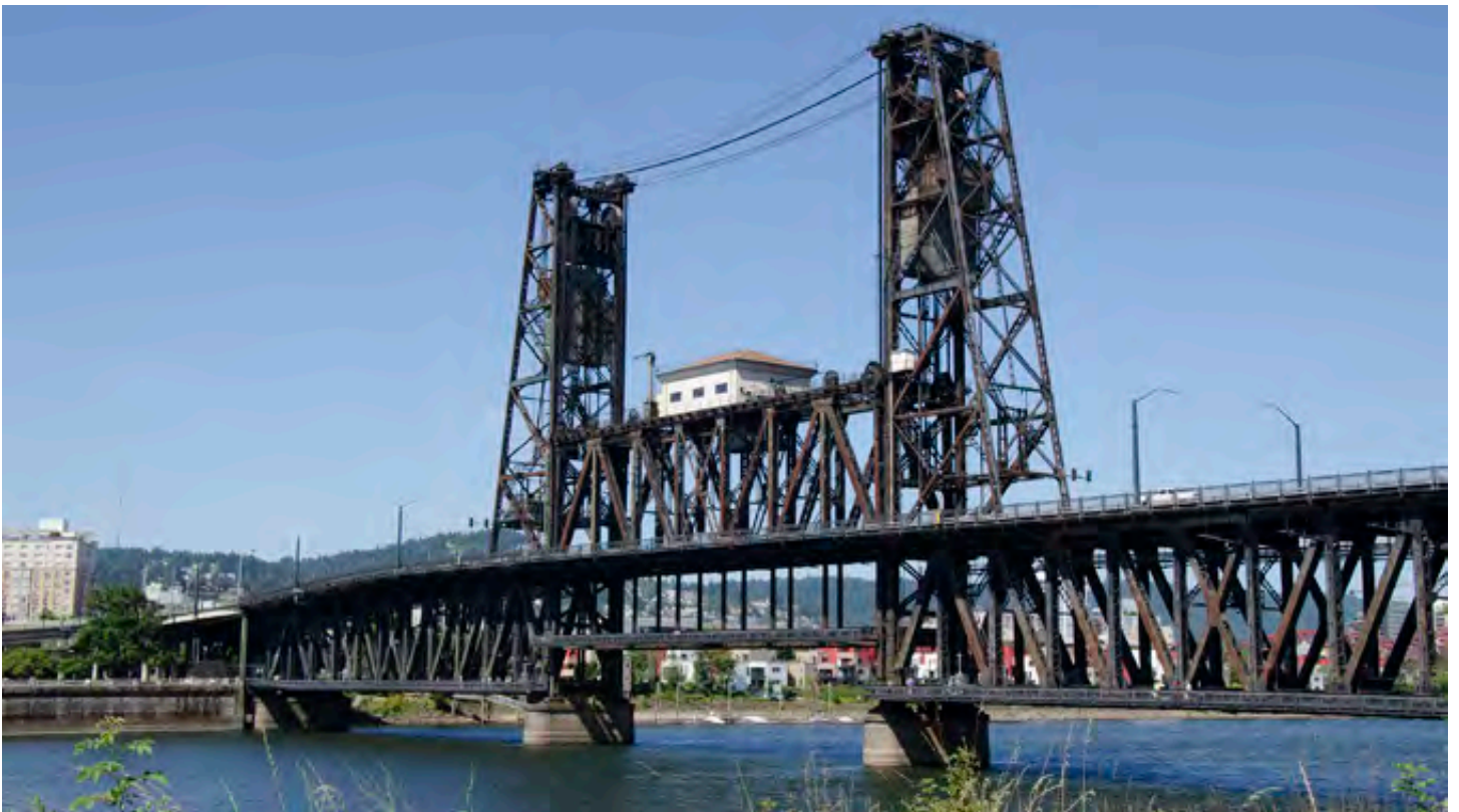
The Steel Bridge from the Eastbank Esplanade
