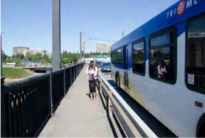
Viewpoint on Steel Bridge north side east of center
