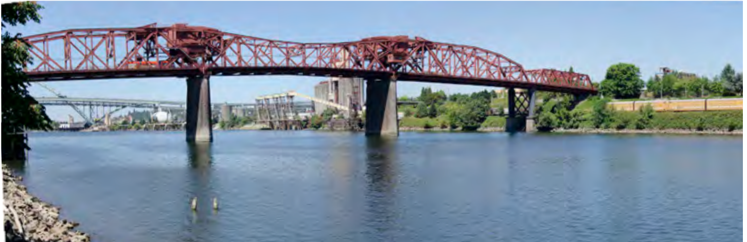
The Broadway Bridge from the Greenway Trail (west)
