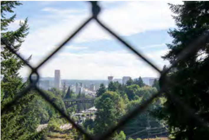
Vista Avenue Viaduct from SW Sherwood Boulevard
