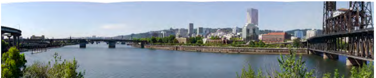
View from mid-ramp on the bike/ped path south of Steel Bridge
