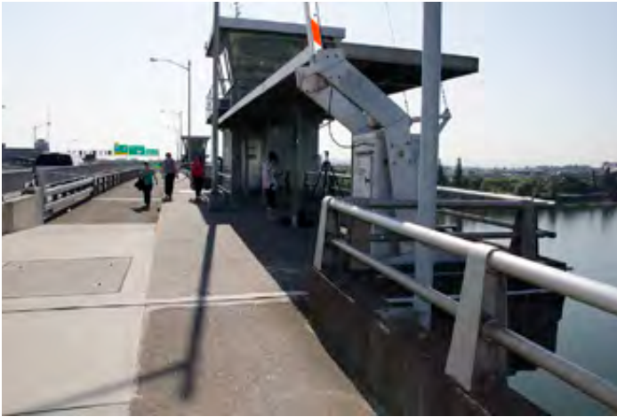
Viewpoint on Morrison Bridge south side, west bump-out
