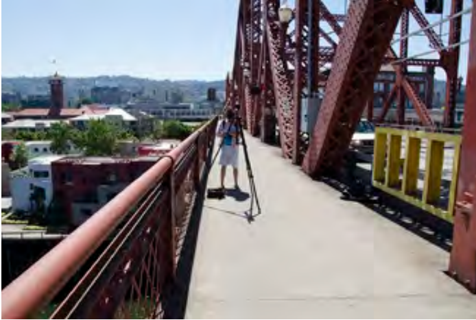
Viewpoint on Broadway Bridge south side west
