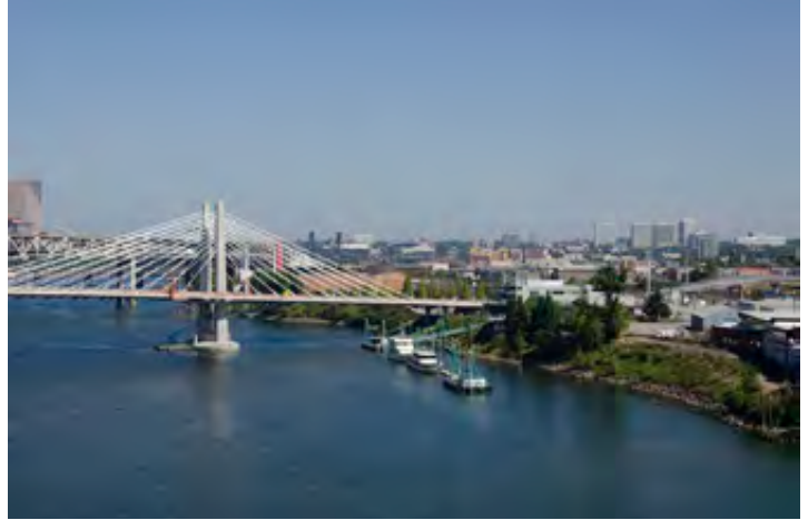
View from Ross Island Bridge north side center, looking north
