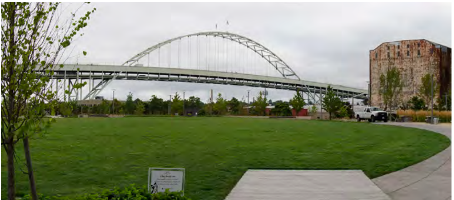
View from The Fields Park southeast path
