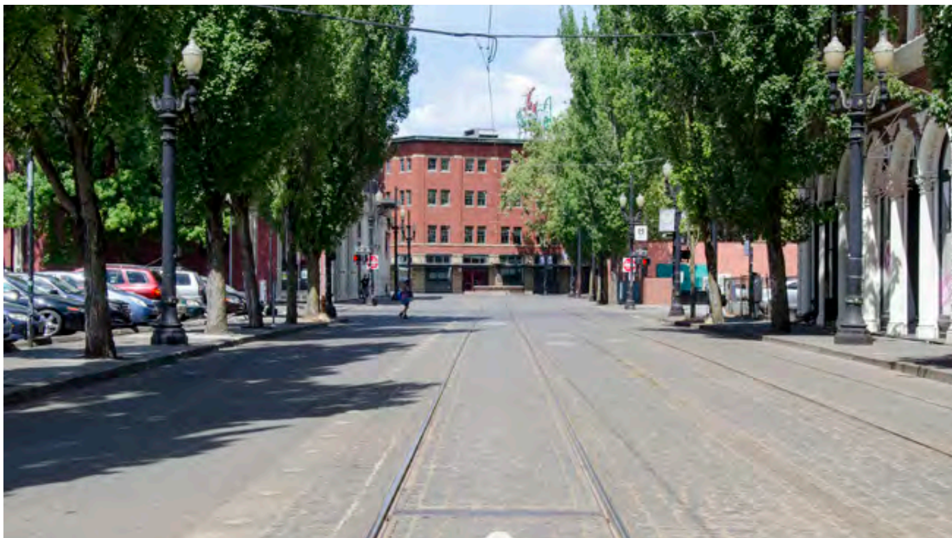
Photo captured east on SW 1st Avenue from SW Pine Street
