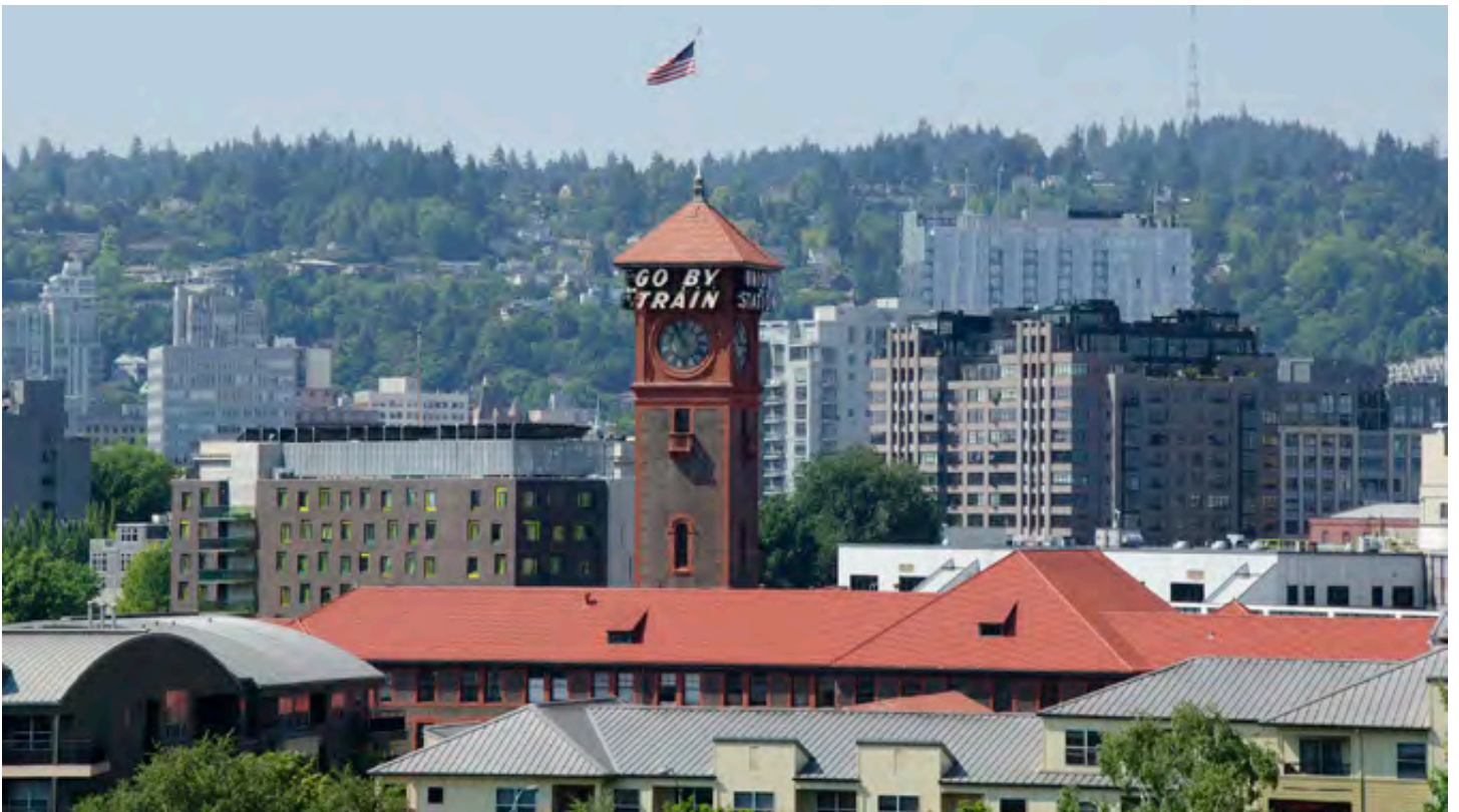
Union Station clock tower from the Broadway Bridge
