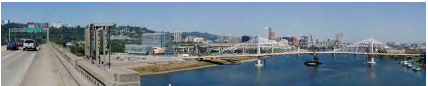
View from Ross Island Bridge north side center, looking north
