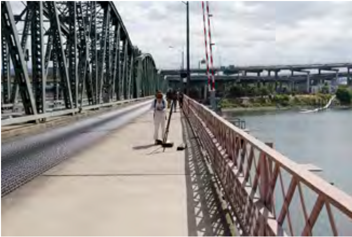
Viewpoint on Hawthorne Bridge south side center
