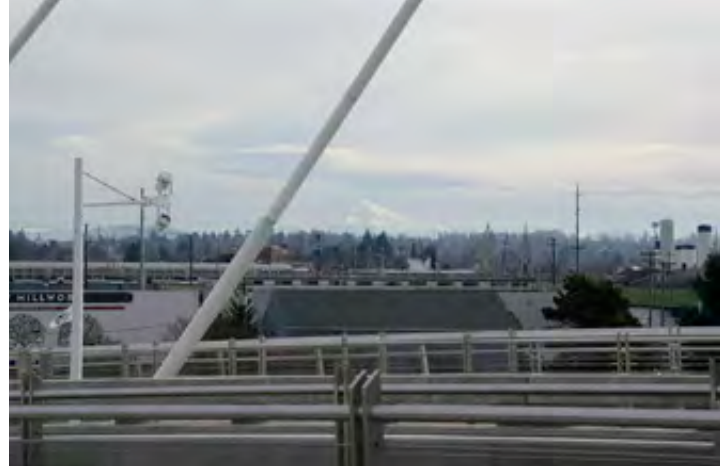
Additional view of Mt Hood from Tilikum Crossing, north side, east bump-out
