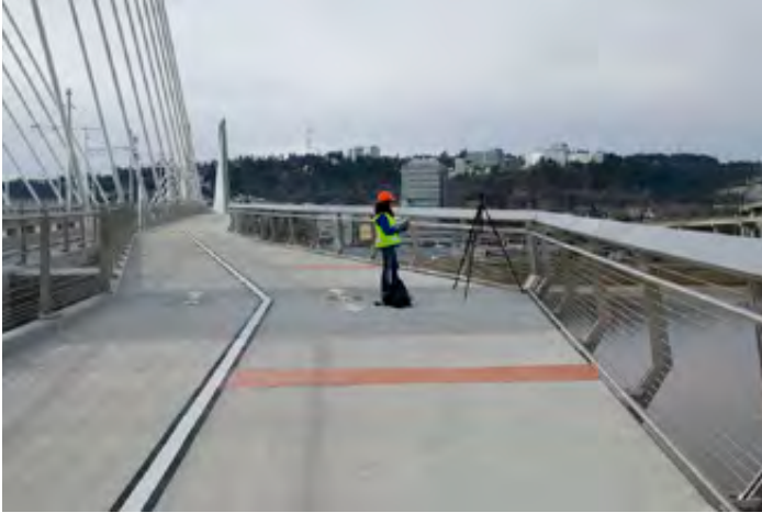
Viewpoint on Tilikum Crossing, north side, east bump-out
