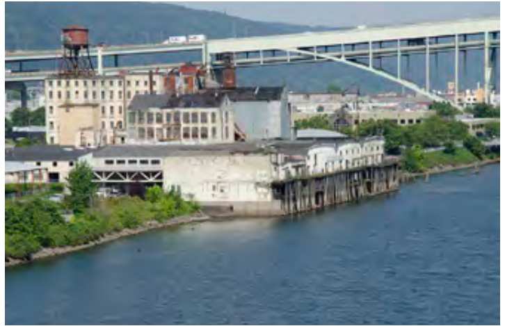
Photo Caption View from Broadway Bridge north side center
