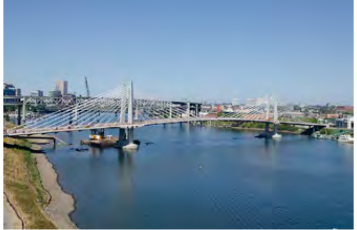
View from Ross Island Bridge north side west of center
