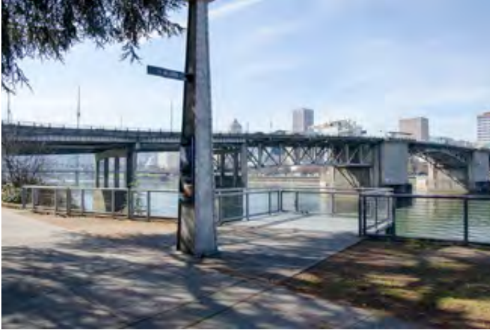
Viewpoint along Eastbank Esplanade at SE Alder Street
