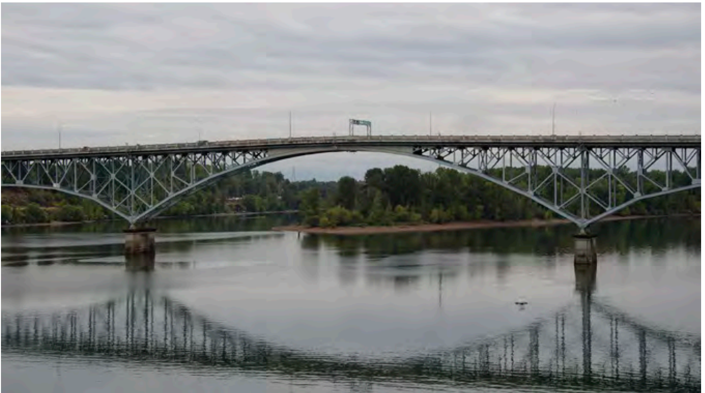
The Ross Island Bridge from Tilikum Crossing
