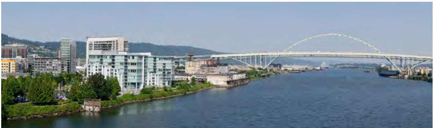
View from Broadway Bridge north side center
