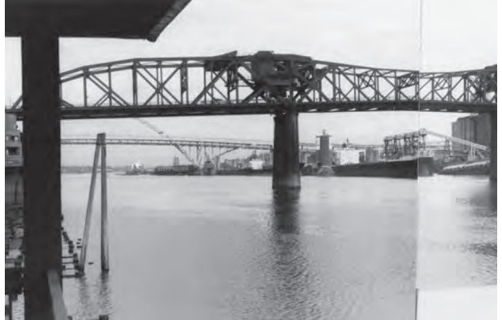
Historic view from Greenway Trail between Broadway and Steel Bridges
