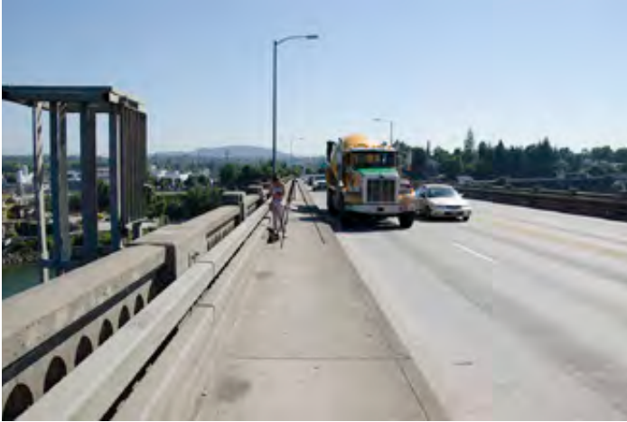
Viewpoint on Ross Island Bridge north side center
