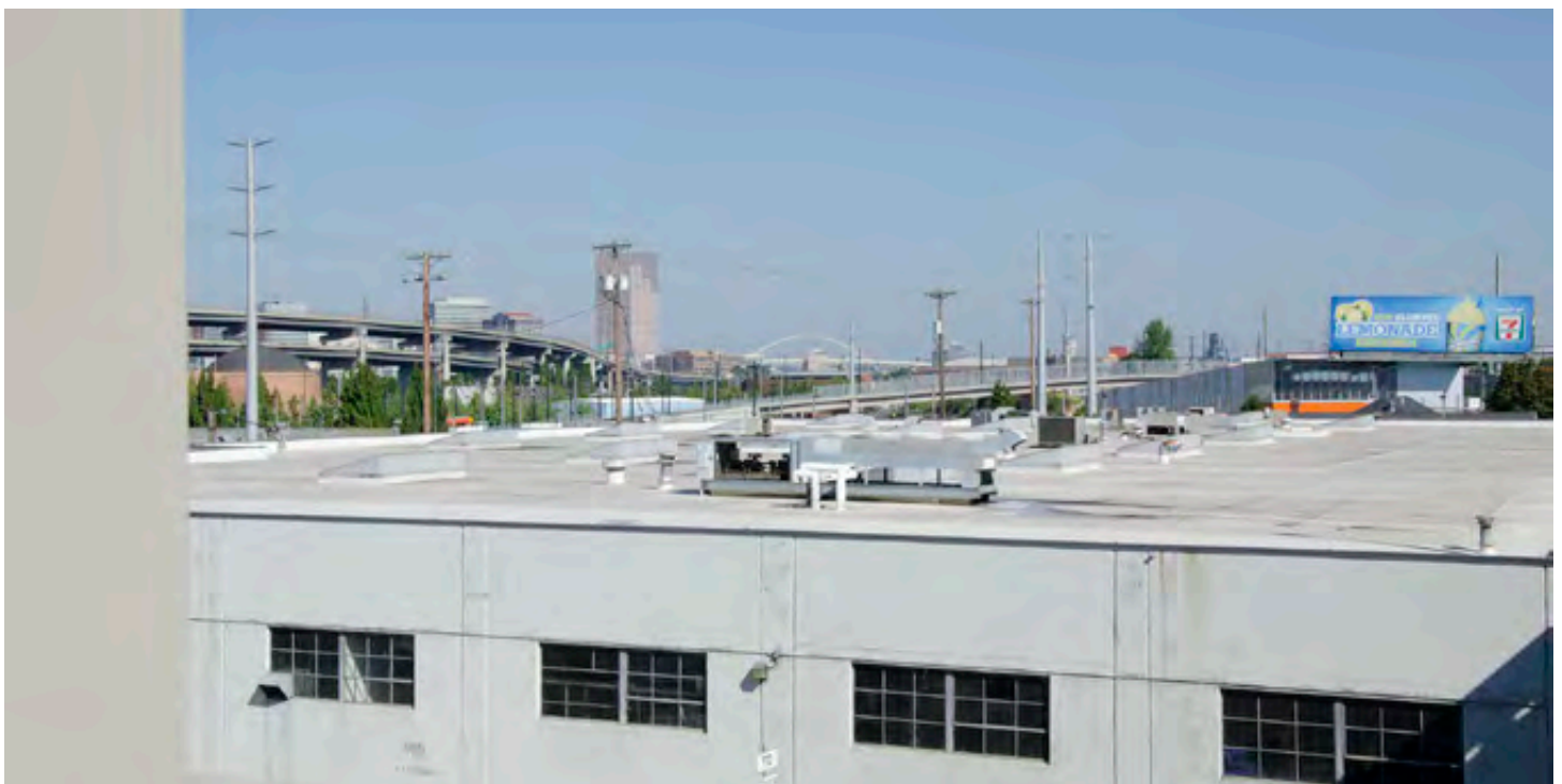
View from MLK Viaduct above SE Division Place, looking north
