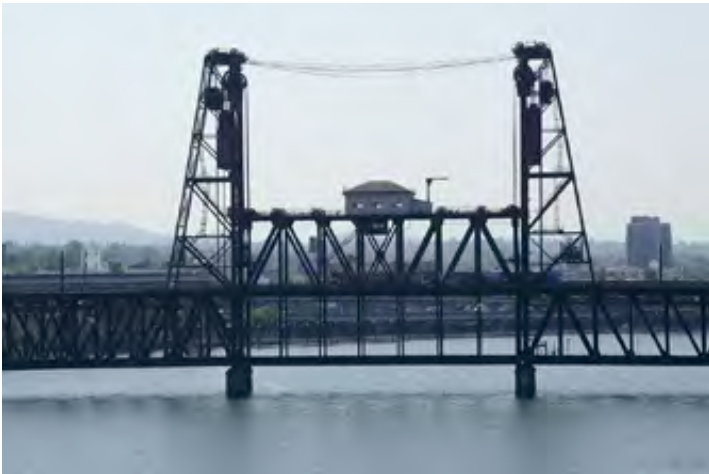
The Steel Bridge from the Broadway Bridge
