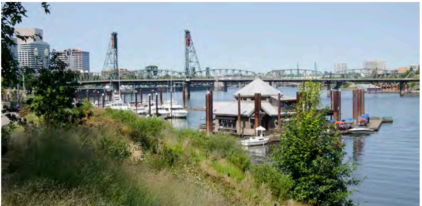
View from Greenway Trail at south end of gardens by SW Montgomery Street, looking north
