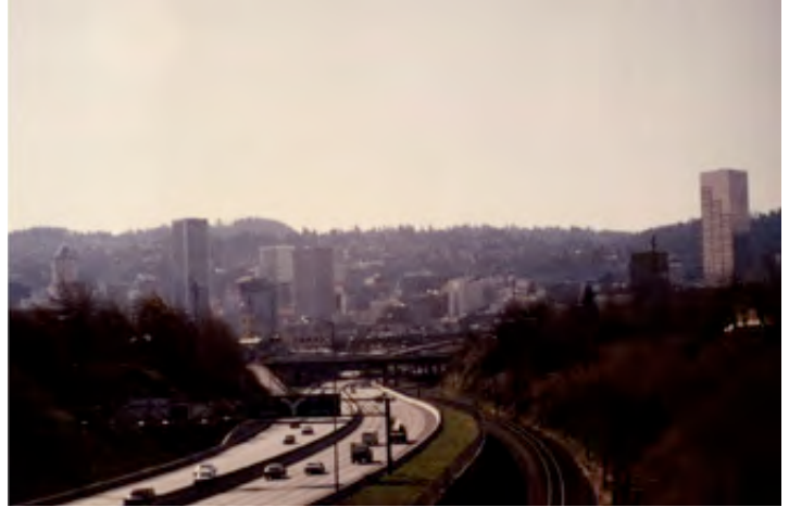
Historic view from NE 12th Avenue I-84 overpass
