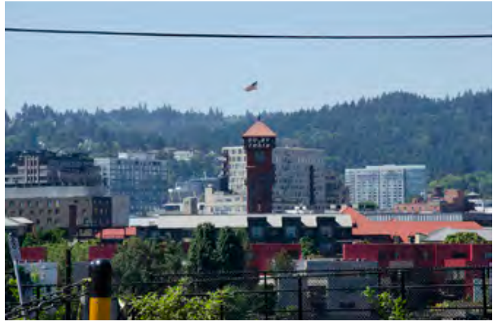
View of Union Station from N Larrabee and N Interstate Avenues
