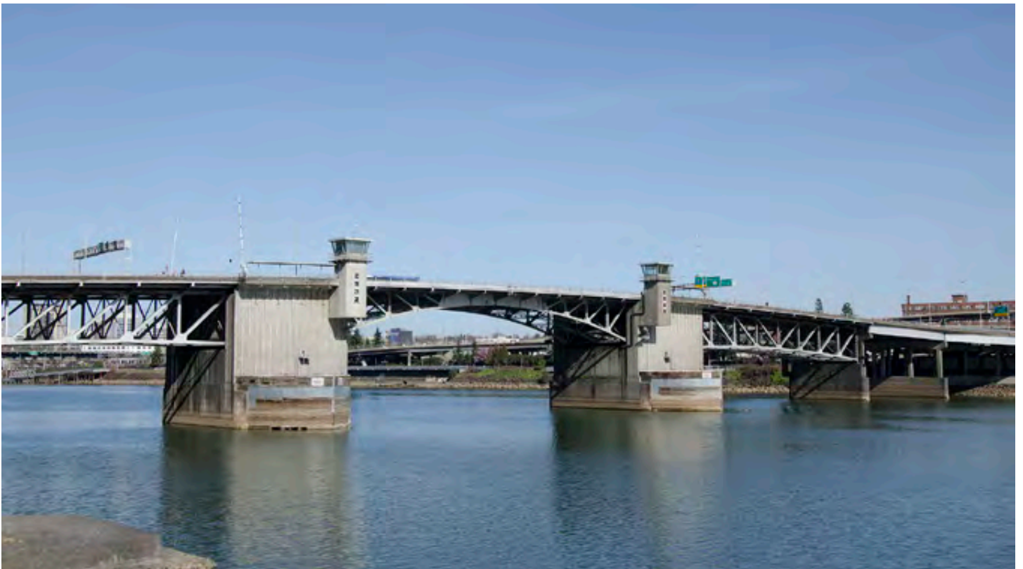
The Morrison Bridge from the Greenway Trail (west)
