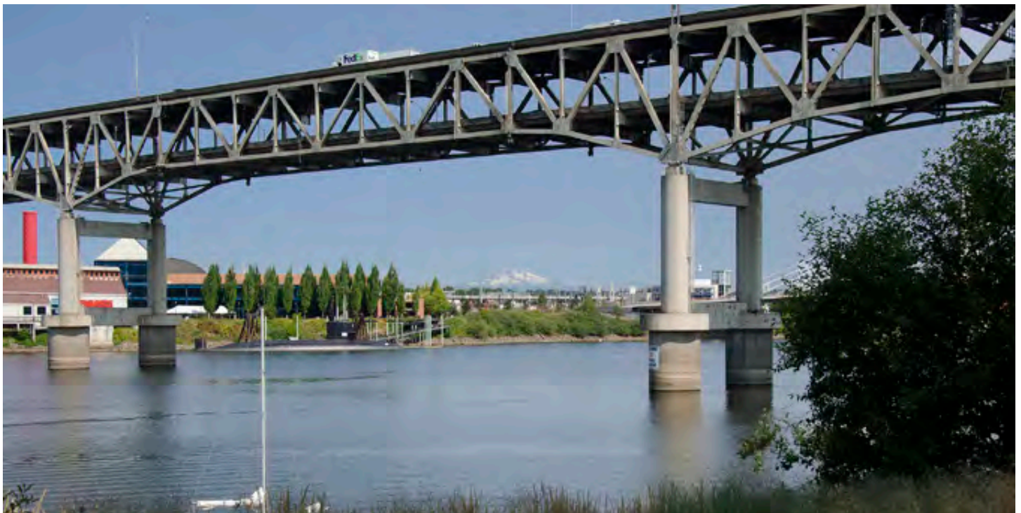
View from Greenway Trail between SW Montgomery Street and SW Hall Street
