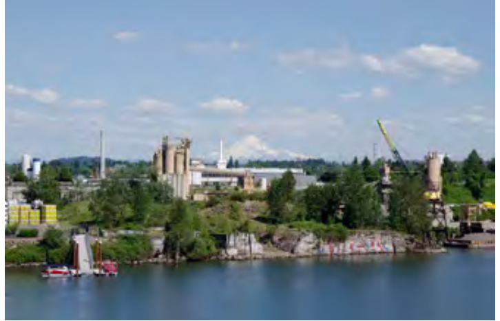
View from Tilikum Crossing, south side, west bump-out
