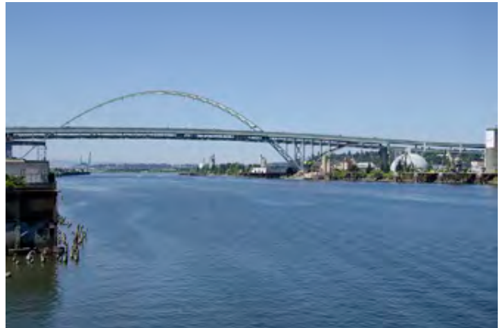
The Fremont Bridge from the Greenway Trail (west)
