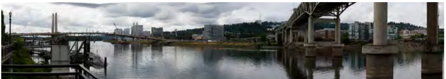
View from Greenway Trail (east) OMSI north viewpoint just south of Marquam Bridge
