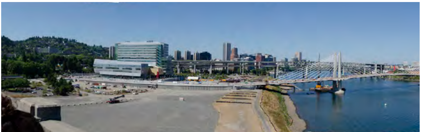
View from Ross Island Bridge north side west of center
