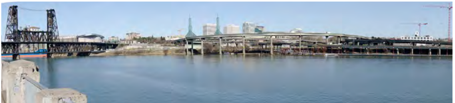
View from Greenway Trail at NW Couch Street
