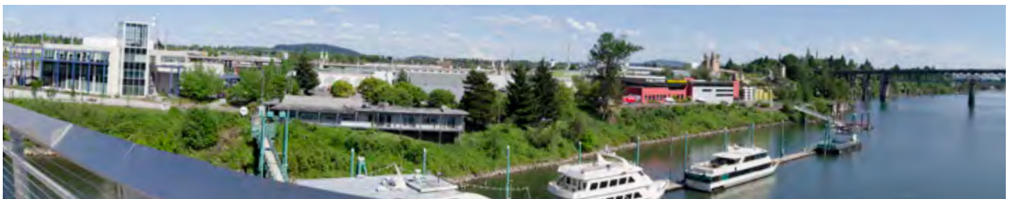
View from Tilikum Crossing, south side, east bump-out
