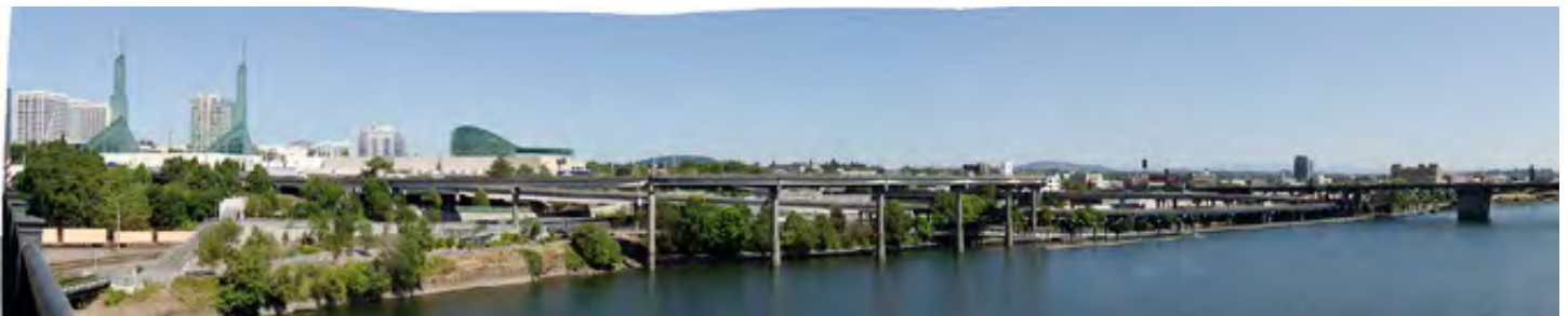
View from Steel Bridge upper deck, south side center
