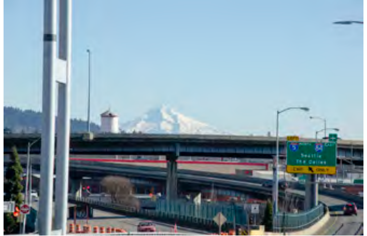
Additional view of Mt Hood from Morrison Bridge south side east bump-out
