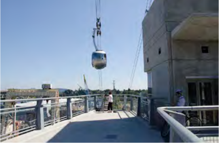
View from SW Gibbs Street pedestrian bridge
