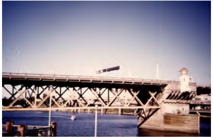
Historic view from Greenway Trail at SW Ankeny Street
