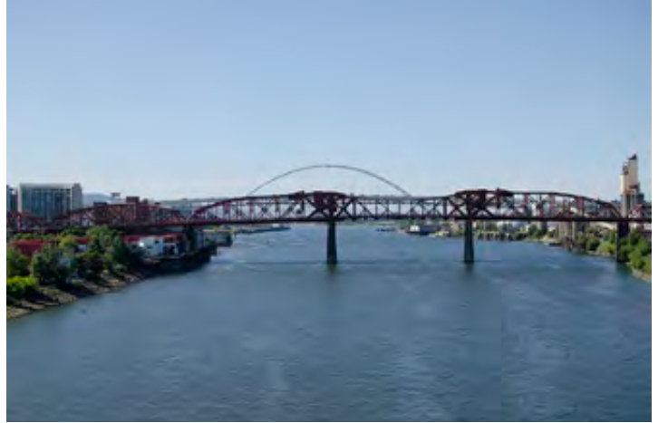
View from Steel Bridge north side center
