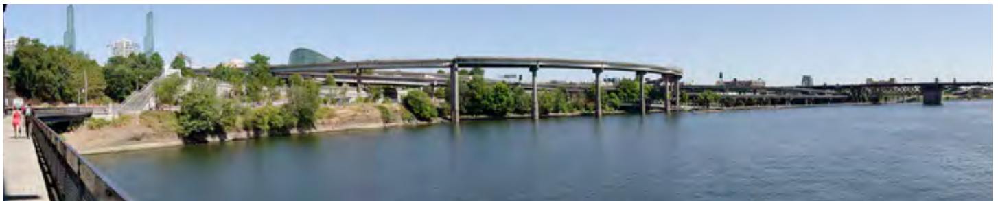
View from Steel Bridge lower deck bike/pedestrian path
