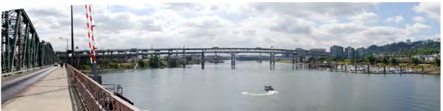
View from Hawthorne Bridge south side center
