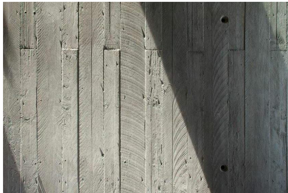
BOARD FORMED CONCRETE
