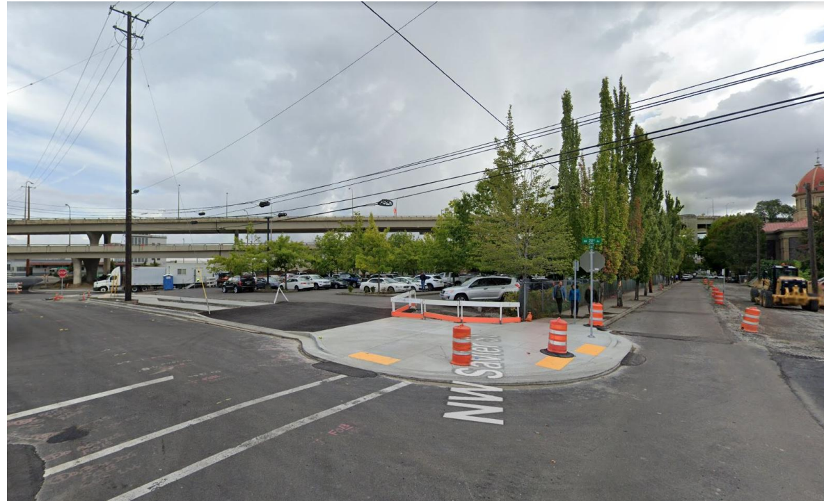
BLOCK 261 FROM SOUTHWEST
