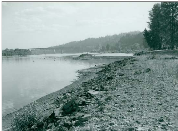
Historic photo of view of the original Sellwood Bridge from the western shore of the Willamette River.
