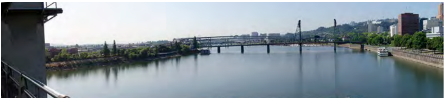
View from Morrison Bridge south side, west bump-out
