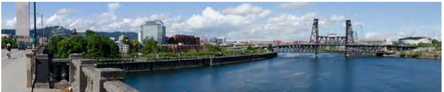
View from Burnside Bridge north side center
