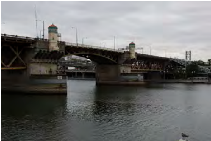
The Burnside Bridge from the Greenway Trail (west)
