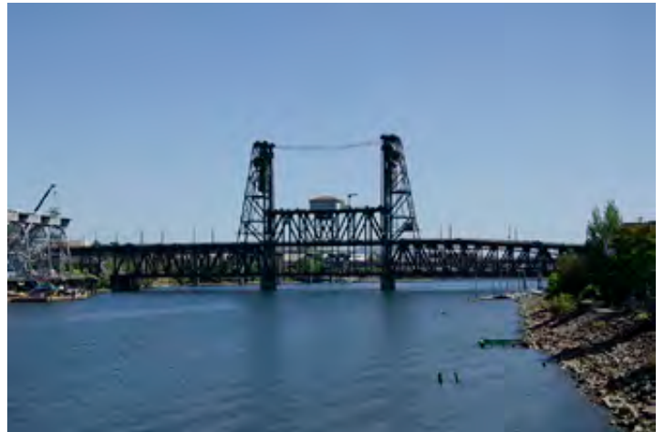
The Steel Bridge from the Greenway Trail (west)
