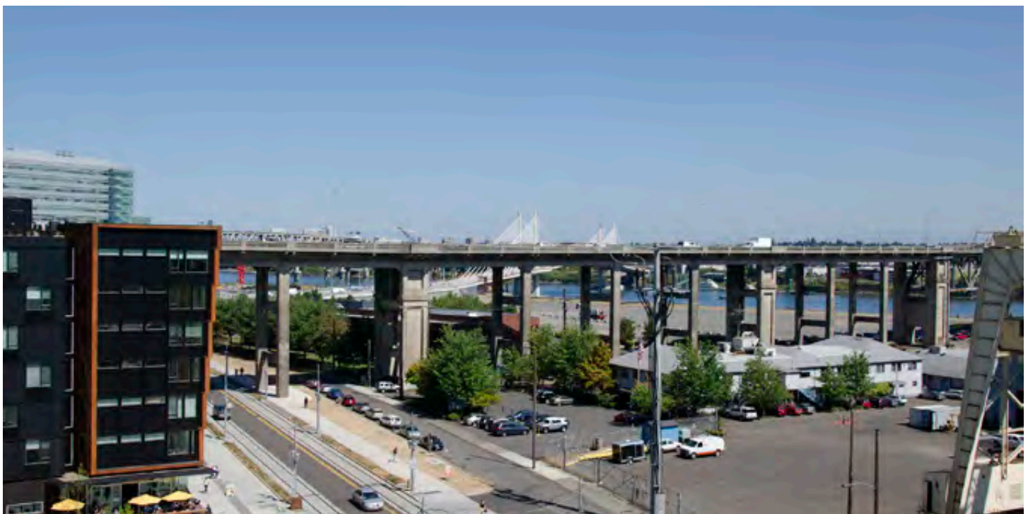
View from SW Gibbs Street pedestrian bridge, looking north
