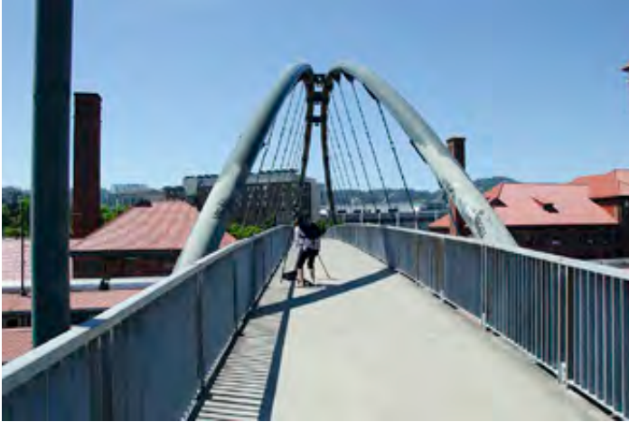
Viewpoint on Union Station pedestrian bridge
