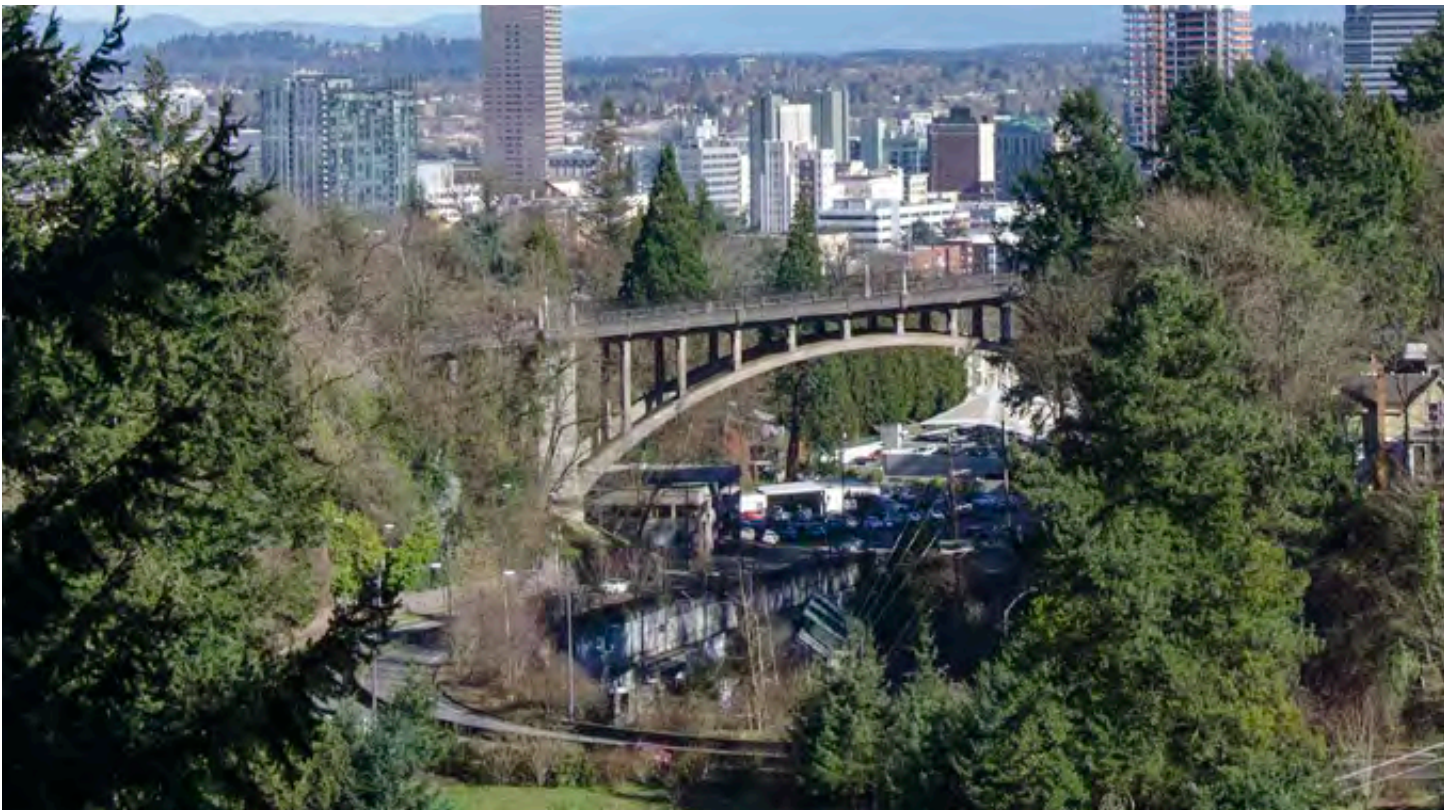
Vista Avenue Viaduct from SW Sherwood Boulevard
