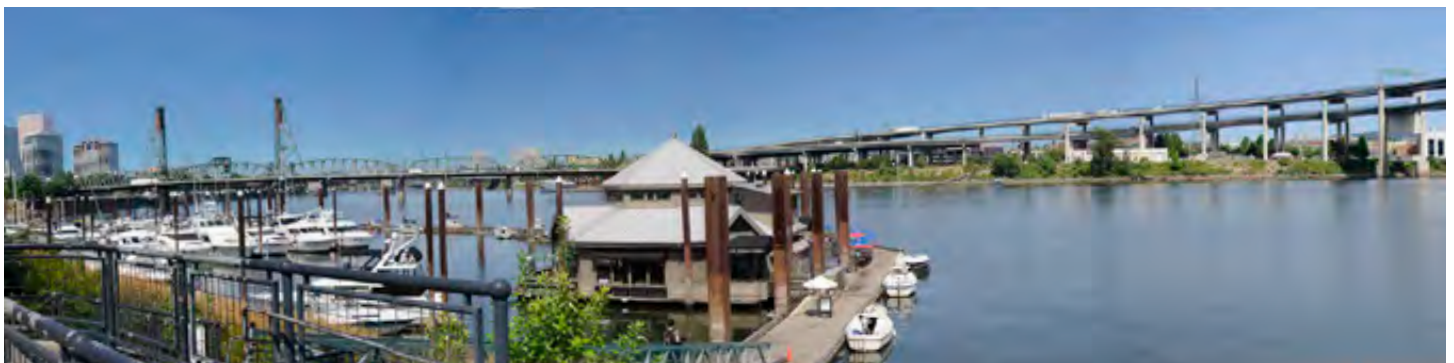
View from Greenway Trail south of Riverplace south public dock
