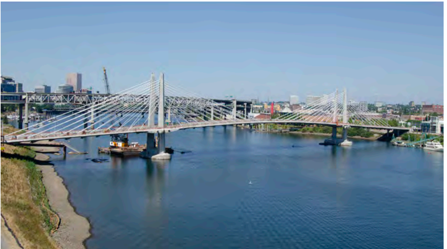
Tilikum Crossing from the Ross Island Bridge
