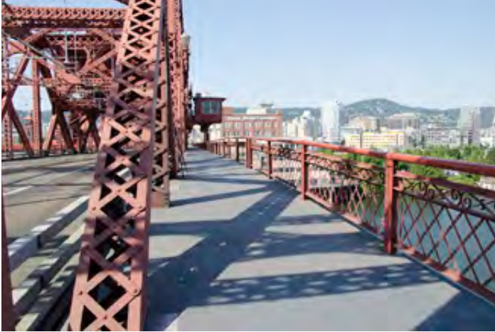
Viewpoint on Broadway Bridge north side center
