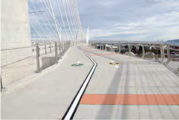
Viewpoint on Tilikum Crossing, south side, west bump-out
