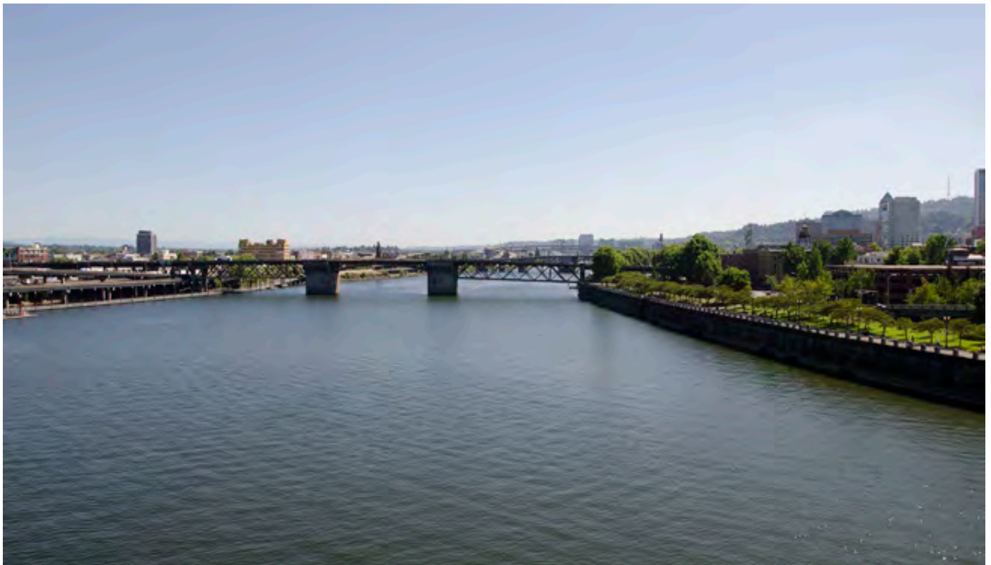
The Willamette River - view from the Steel Bridge
