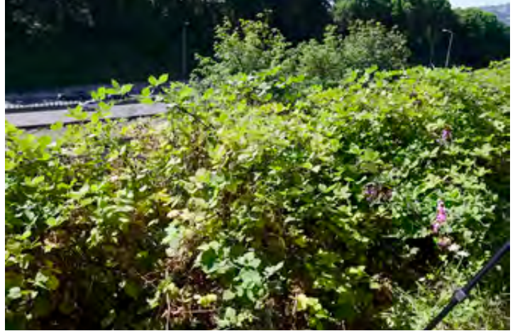
Overgrown vegetation at NE Lloyd Boulevard west of NE 9th Avenue
