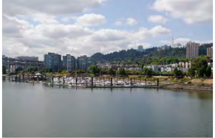
View from Hawthorne Bridge south side center
