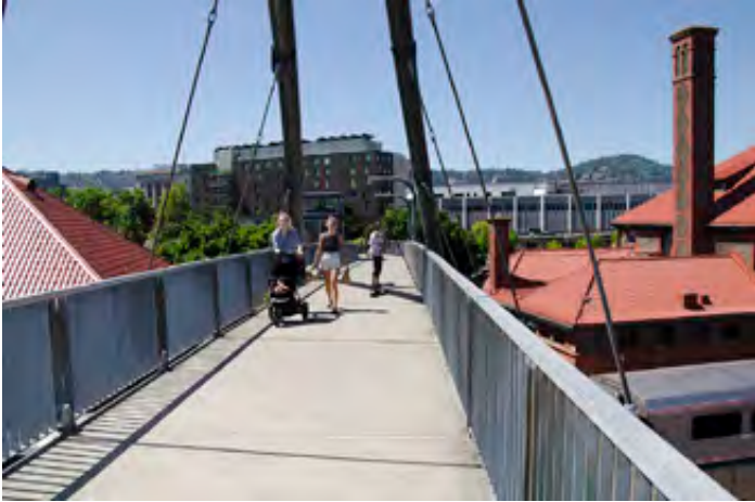
Viewpoint on Union Station pedestrian bridge
