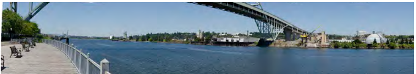
View from Greenway Trail just south of Fremont Bridge
