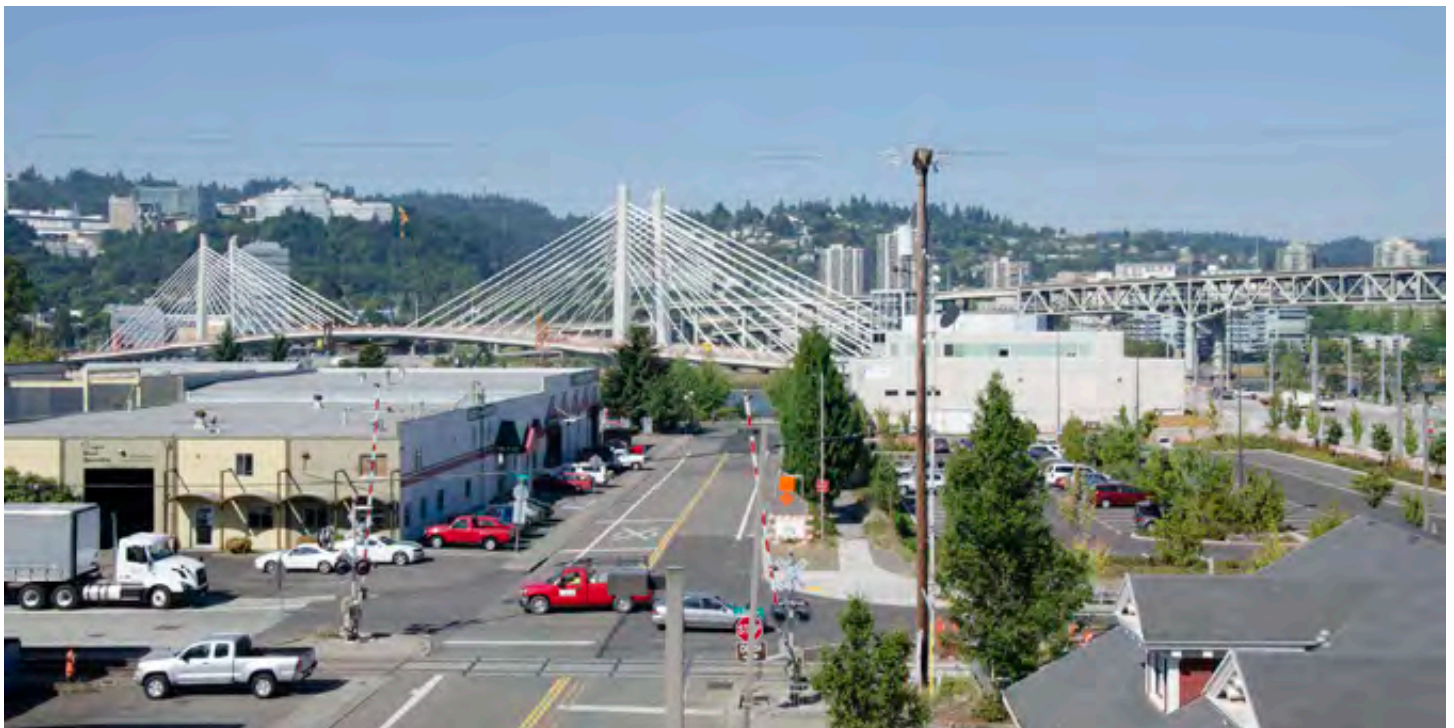
View from MLK Viaduct above SE Caruthers Street
