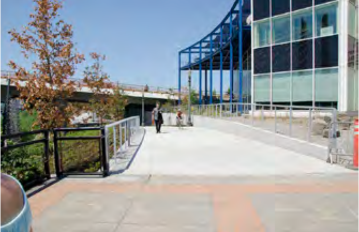
Greenway Trail (east) at SE Caruthers Street
