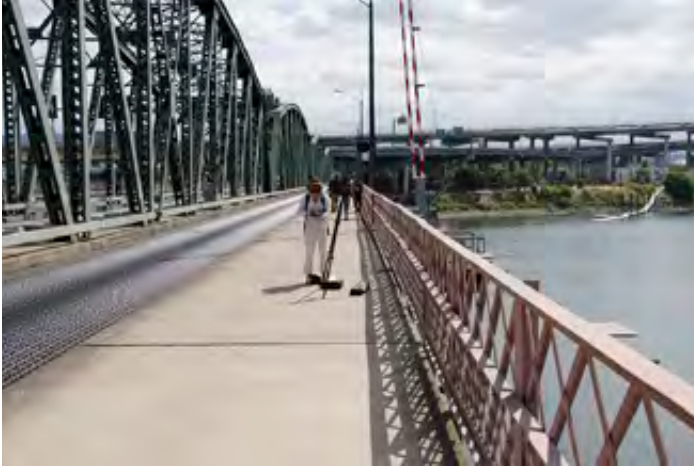
Viewpoint on Hawthorne Bridge south side center
