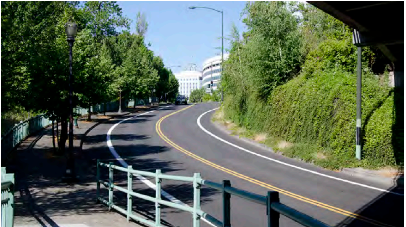
Looking west from NE 16th Avenue under I-84 ramp
