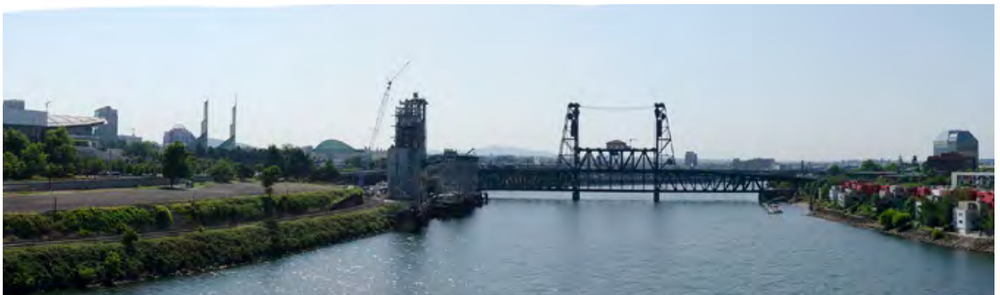
View from Broadway Bridge south side center
