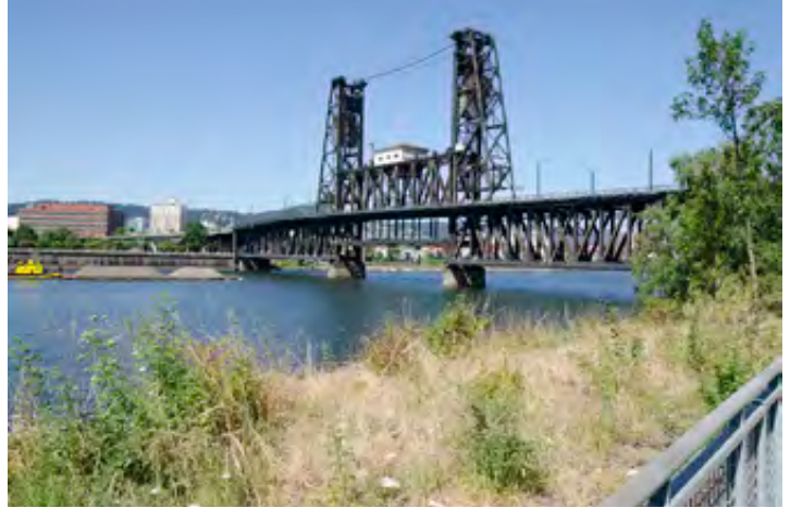
View of Steel Bridge from Eastbank Esplanade south of Steel Bridge
