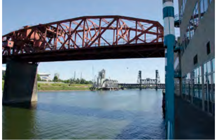
View from Greenway Trail just north of Broadway Bridge
