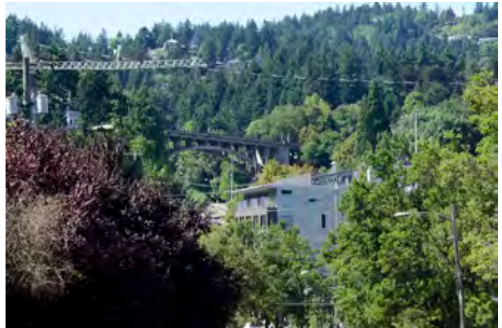
Vista Avenue Viaduct from SW Jefferson Street and SW 14th Avenue
