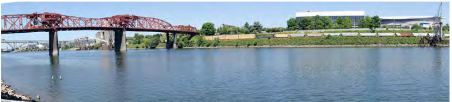
View from Greenway Trail between Broadway and Steel Bridges
