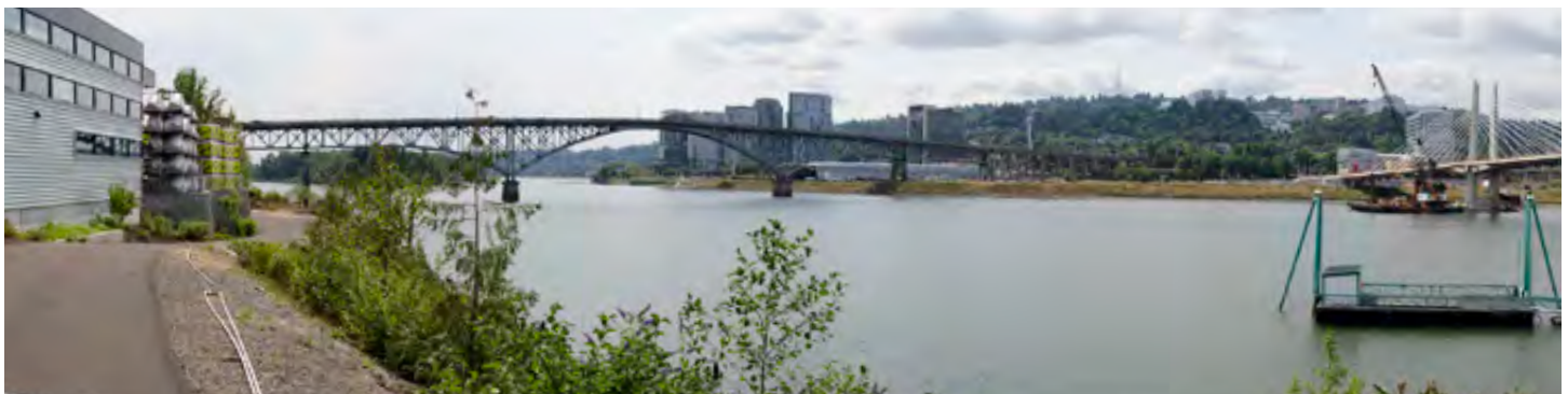
View from Greenway Trail (east) between SE Division Place and SE Ivon Street
