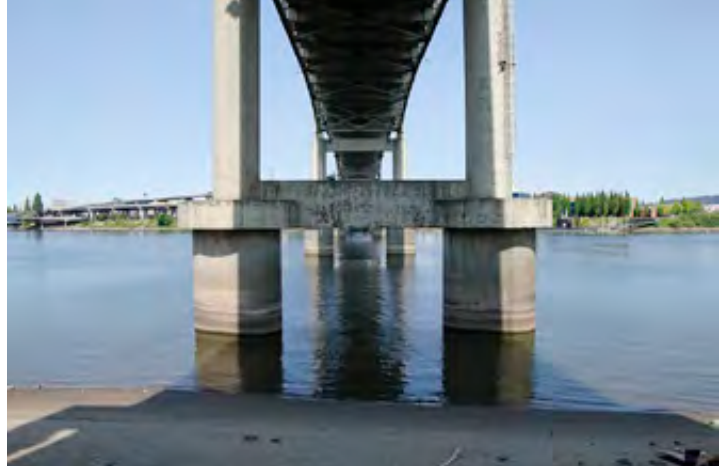
View from Greenway Trail under Marquam Bridge
