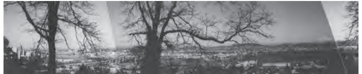
Historic view from SW Terwilliger Boulevard north of SW Condor Lane
