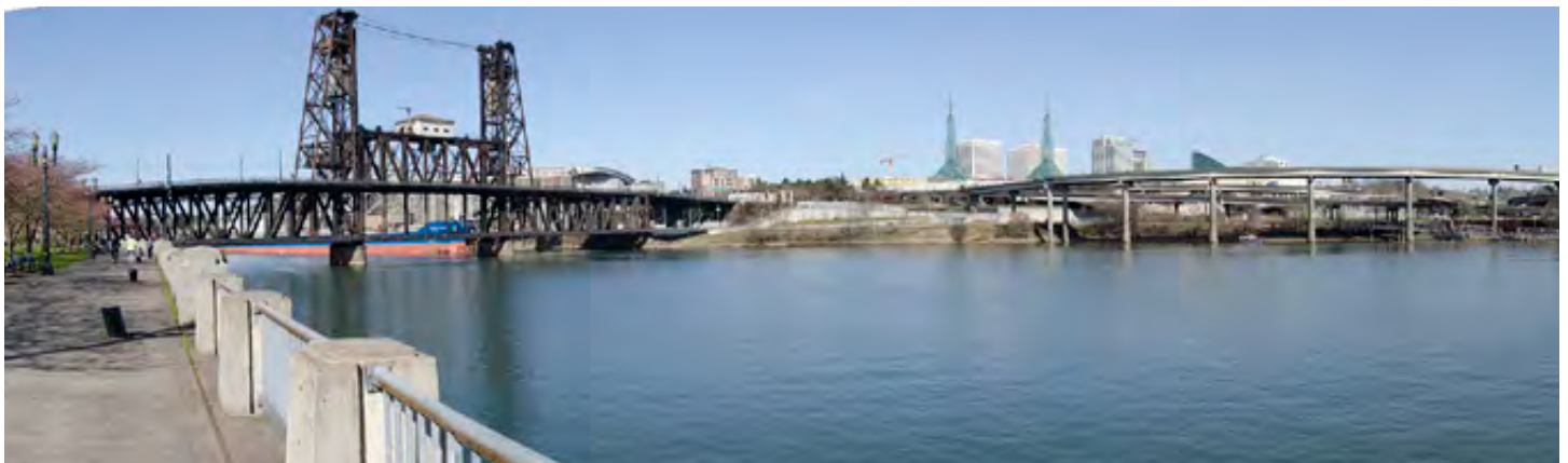
View from Greenway Trail West at stairs near NW Everett Street
