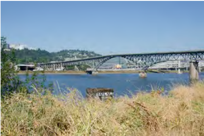
The Ross Island Bridge from Springwater Corridor
