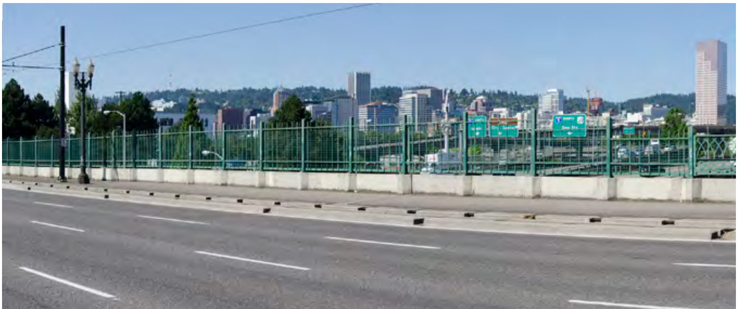
View from NE MLK Jr Boulevard and Interstate 84 overpass
