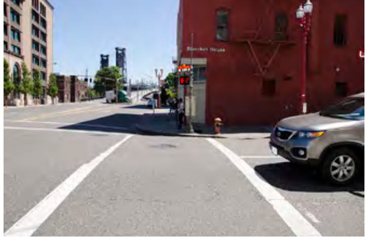
View of Steel Bridge from NW Glisan Street and NW 4th Avenue
