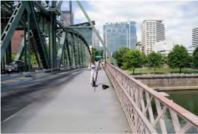
Viewpoint on Hawthorne Bridge north side west of center
