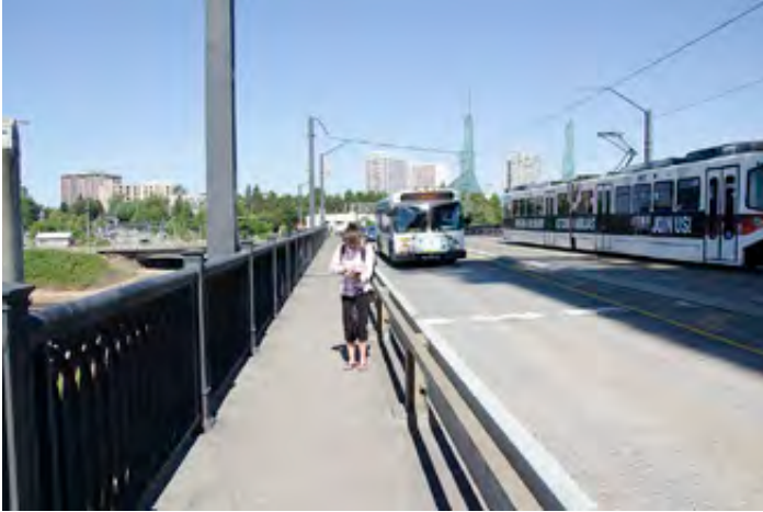
Viewpoint on Steel Bridge north side center
