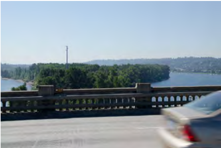
Ross Island from the Ross Island Bridge
