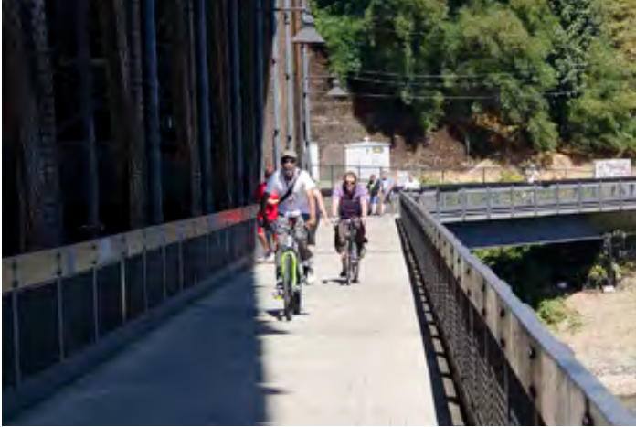
Viewpoint along Steel Bridge lower deck bike/pedestrian path
