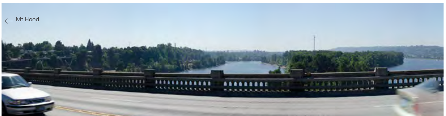
View from Ross Island Bridge north side center, looking south
