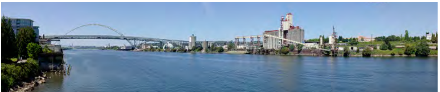
View from Greenway Trail just north of Broadway Bridge
