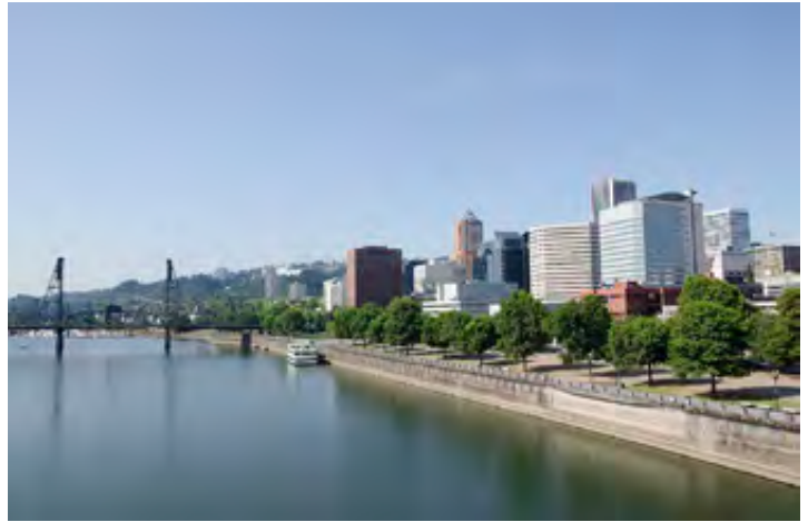
View from Morrison Bridge south side, west bump-out
