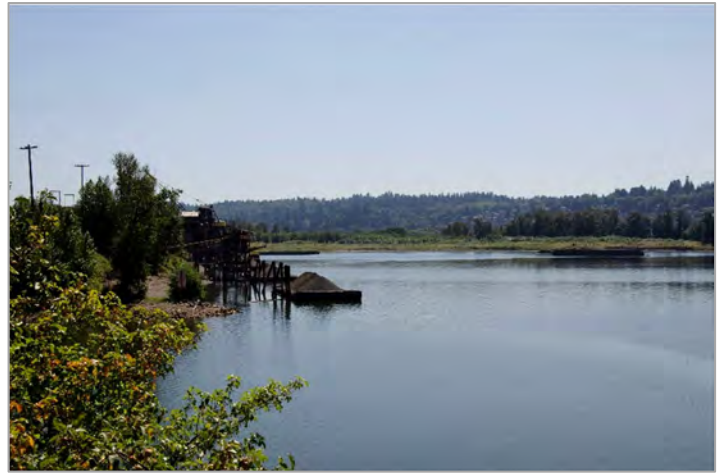
Ross Island Sand and Gravel facilities visible from the viewpoint.
