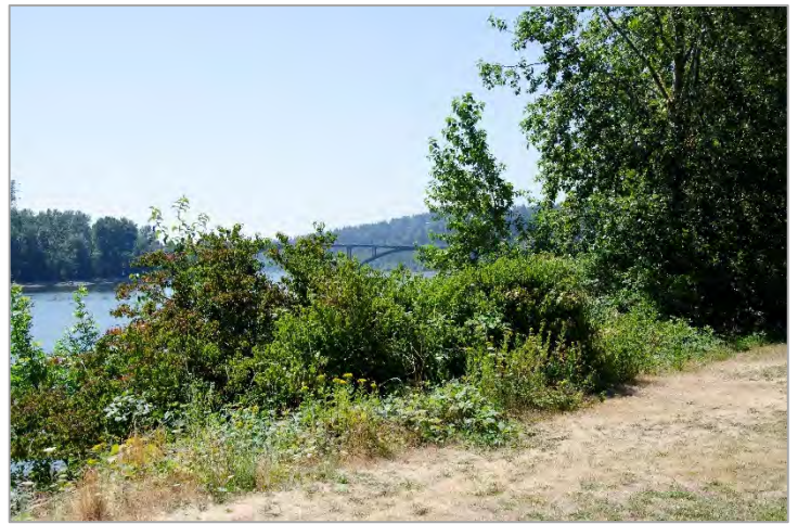
View of Sellwood Bridge partially obscured by vegetation.
