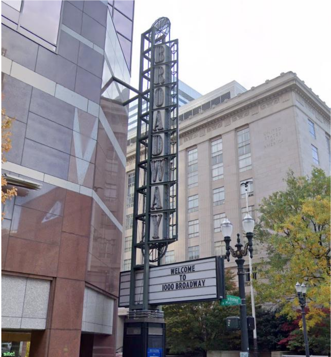
SW BROADWAY AVE. at SW MAIN ST. DECEMBER 2020 BROADWAY THEATER SIGNAGE, MARQUEE and PEDESTAL
