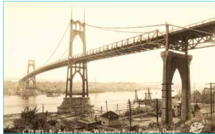
St. Johns Bridge, 1937
