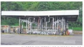
PHOTOS COURTESY OF CARSON OIL CO. Carson Oil Co.'s new \$2 million rack mixes biofuel with petroleum-based fuel as the fuel is transferred into a tanker truck at a rate of 1,163 gallons per minute.
