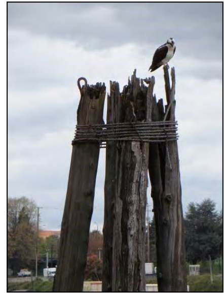
Osprey perched on derelict piling.
