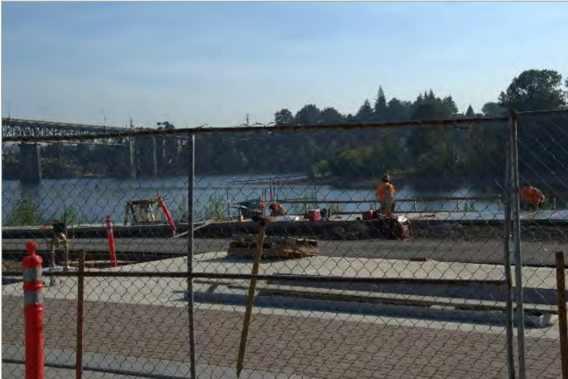
Example: Construction fencing (note: photo taken outside of the South Reach)
