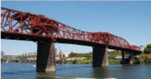
Broadway Bridge, Oregon
