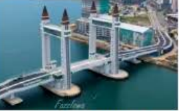
Tereganu Bridge, Malaysia
