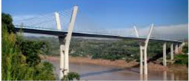
Chongqing Expressway Bridge, Oregon
