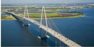
Copper River Bridge, South Carolina
