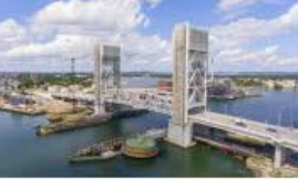
Fore River Bridge, Massachusetts
