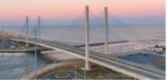
Indian River Inlet Bridge, Delaware
