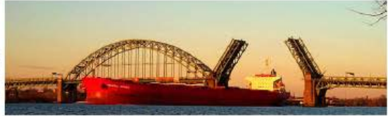
Tacony-Palmyra Bridge, Pennsylvania
