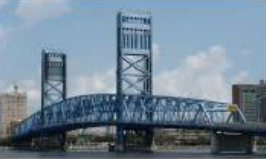
Main Street Bridge, Florida
