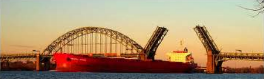
Tacony-Palmyra Bridge, Pennsylvania
