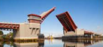
South Park Bridge, Washington
