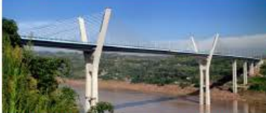
Chongqing Expressway Bridge, Oregon
