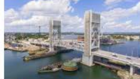
Fore River Bridge, Massachusetts
