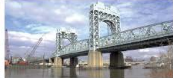
Triborough (Harlem River) Bridge, New York
