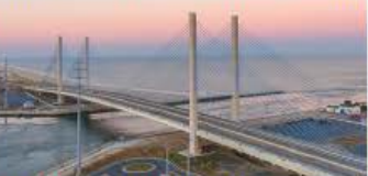
Indian River Inlet Bridge, Delaware
