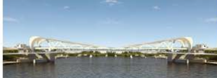
New Johnson St. Bridge, Canada
