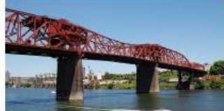
Broadway Bridge, Oregon
