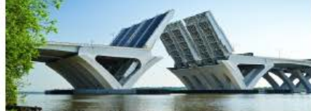
Woodrow Wilson Bridge, Maryland
