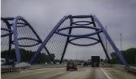
Gateway Bridge, Michigan
