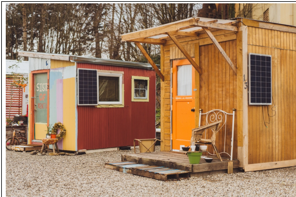
The Kenton Women’s Village An Example of the Outdoor Shelter format.
