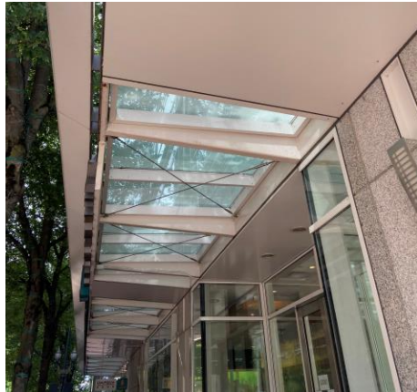
MIST WHITE ALUCOBOND ALUMINUM COMPOSITE METAL CANOPY WITH INTEGRATED ETCHED GLAZING
