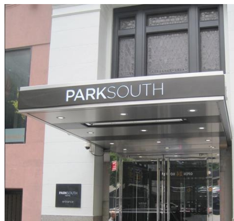
MIST WHITE ALUCOBOND ALUMINUM COMPOSITE METAL CANOPY WITH STATUARY BRONZE HORIZONTAL BANDING
