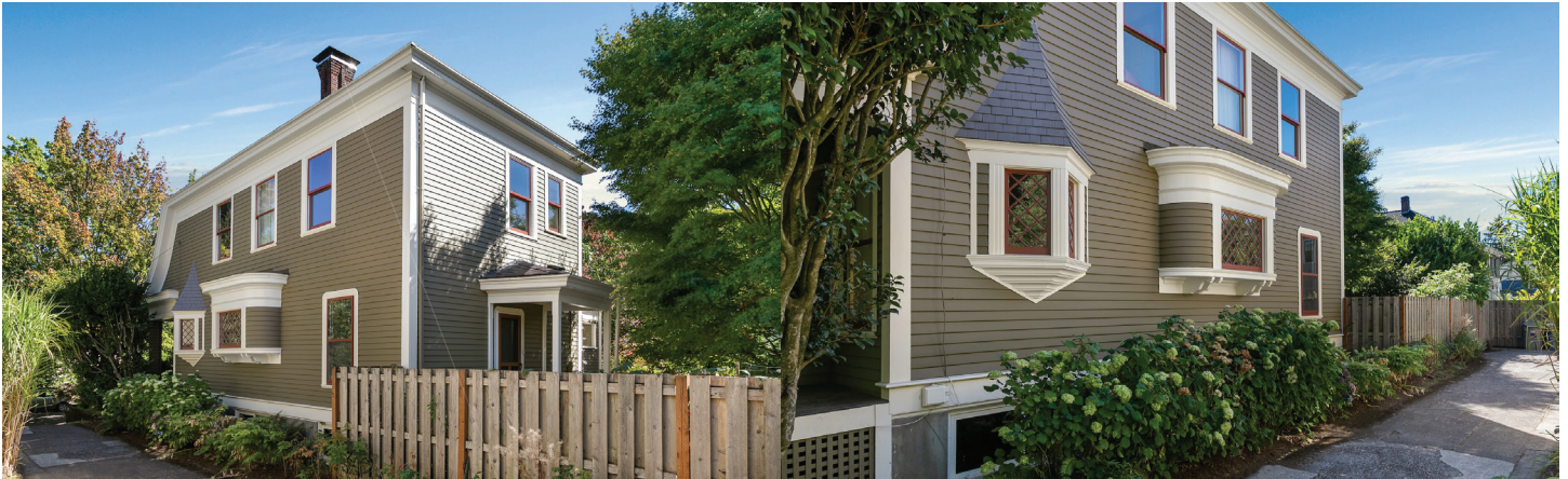
NORTH FACADE FROM SW CORNER
