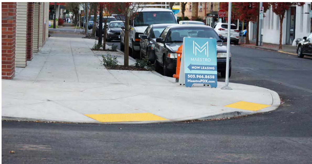
New ADA-compliant curb extensions in Northwest Portland.
