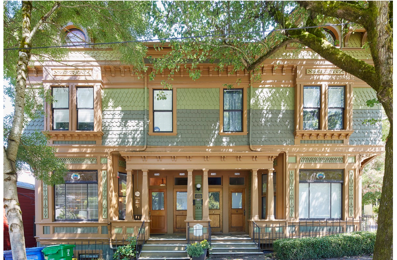
A historic fourplex in the South Portland Historic District
