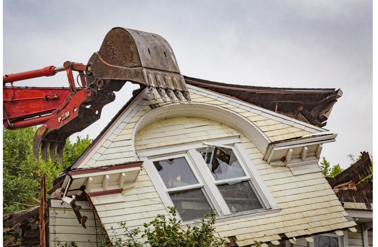
Demolition of a Significant Resource. Photo: Scott Tice.
