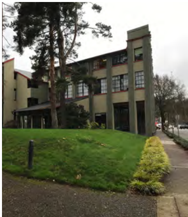
Adaptive reuse of Water Tower building as a commercial business center.
