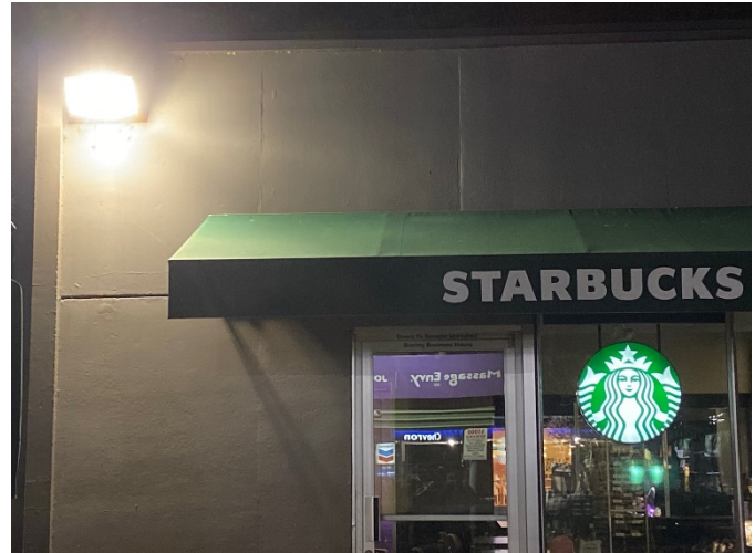
Over-illumination wastes energy and lack of shielding allows light to shine where it is not needed.
