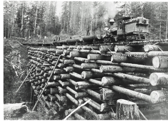
Train trestle bridge constructed of stacked logs
