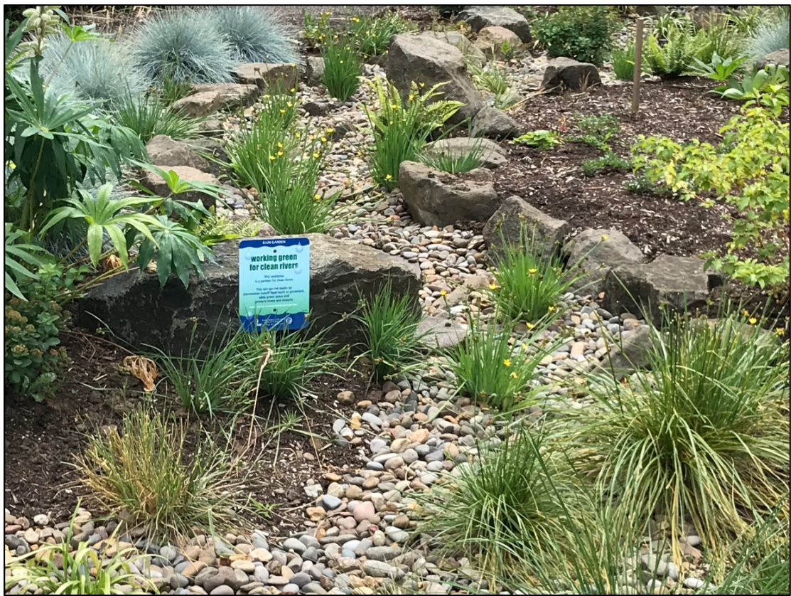
Figure 15 Example retrofit #1, Buckman area rain garden
