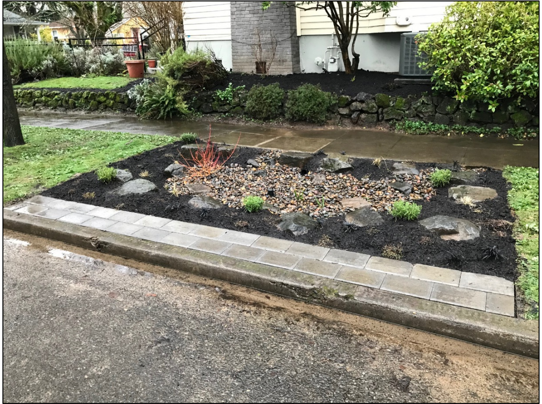
Figure 16 Example retrofit #2, SE Ladd's Right-of-way Rain Garden
