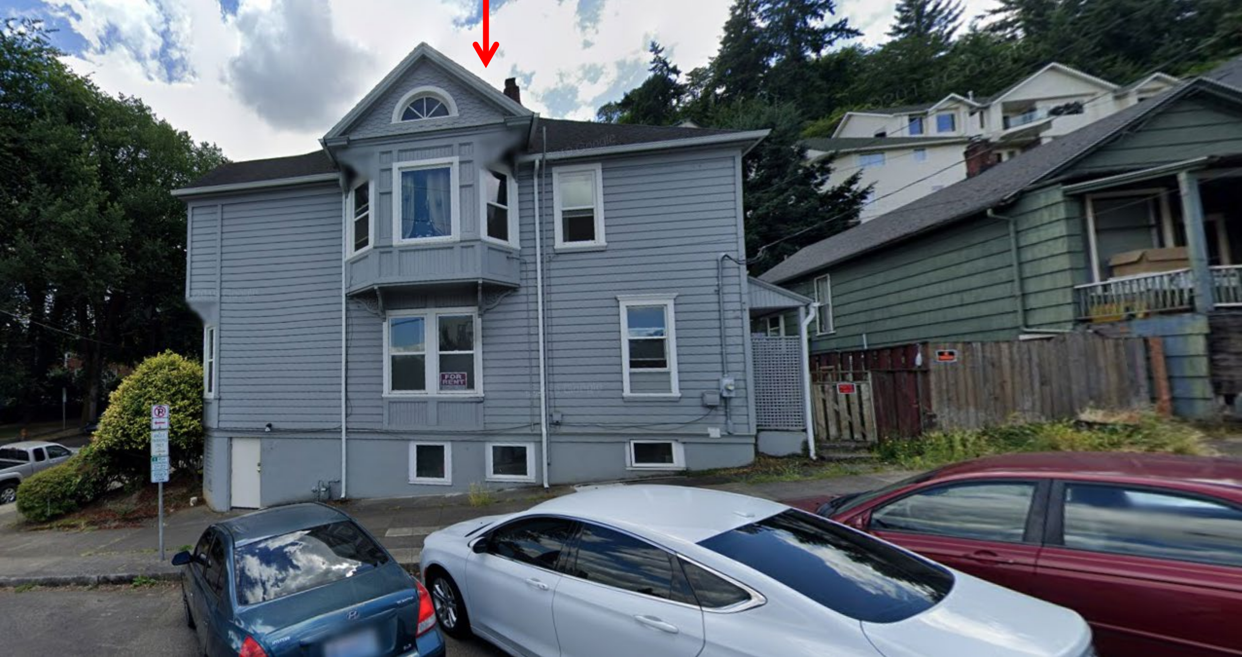
Looking south directly at the site from SW Clifton St
