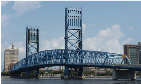
Main Street Bridge, Florida
