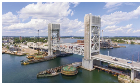
Fore River Bridge, Massachusetts
