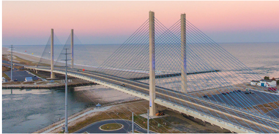
Indian River Inlet Bridge, Delaware
