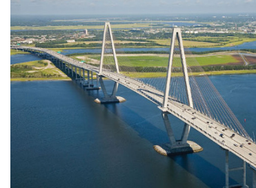
Copper River Bridge, South
