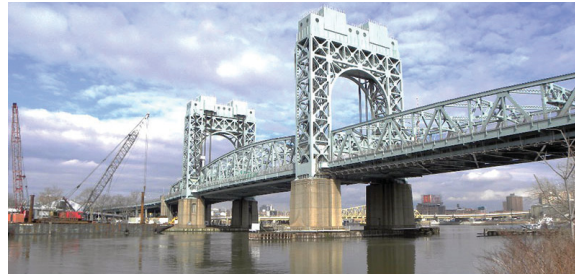
Triborough (Harlem River) Bridge, New York
