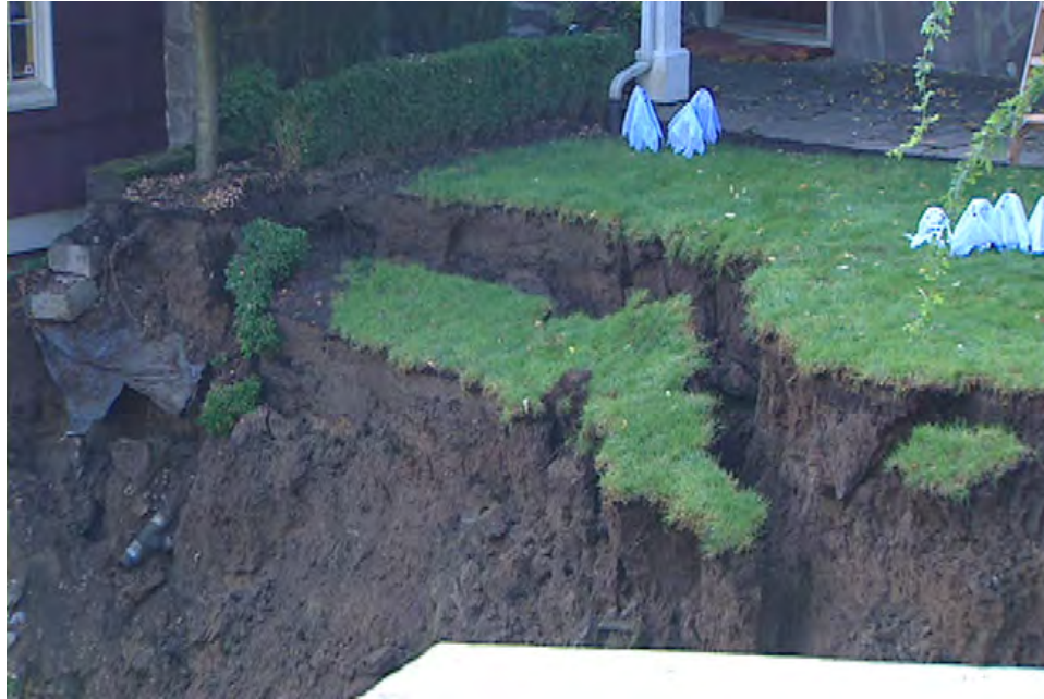
Image: Landslide in Southwest Portland (2008)
