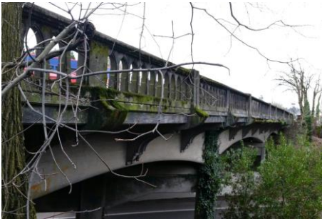
Oregon Electric Railway Overcrossing (replaced)
