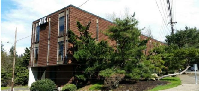
11125 SW Barbur Boulevard (removal)
