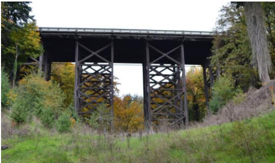
Newbury Viaduct (replaced)
