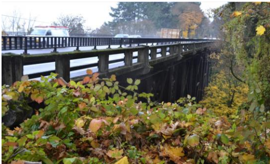
Vermont Viaduct (replaced)
