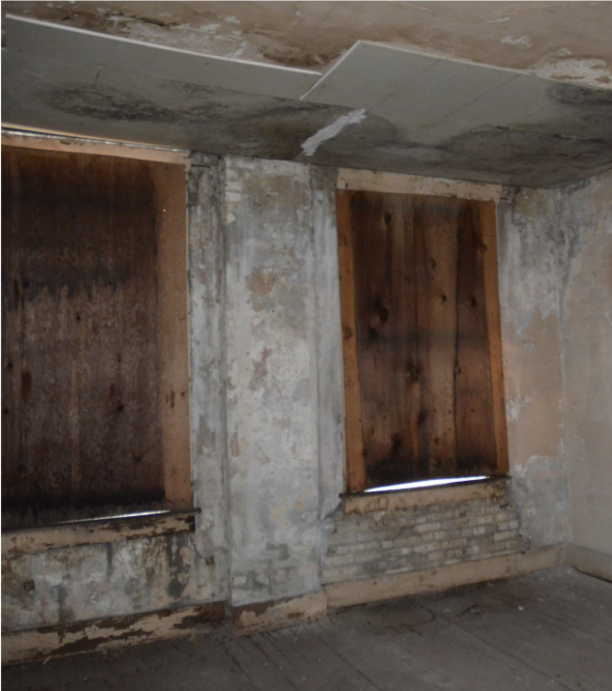
BEFORE: The masonry walls and openings were in extremely poor condition and required full tuck-pointing throughout the interior.
