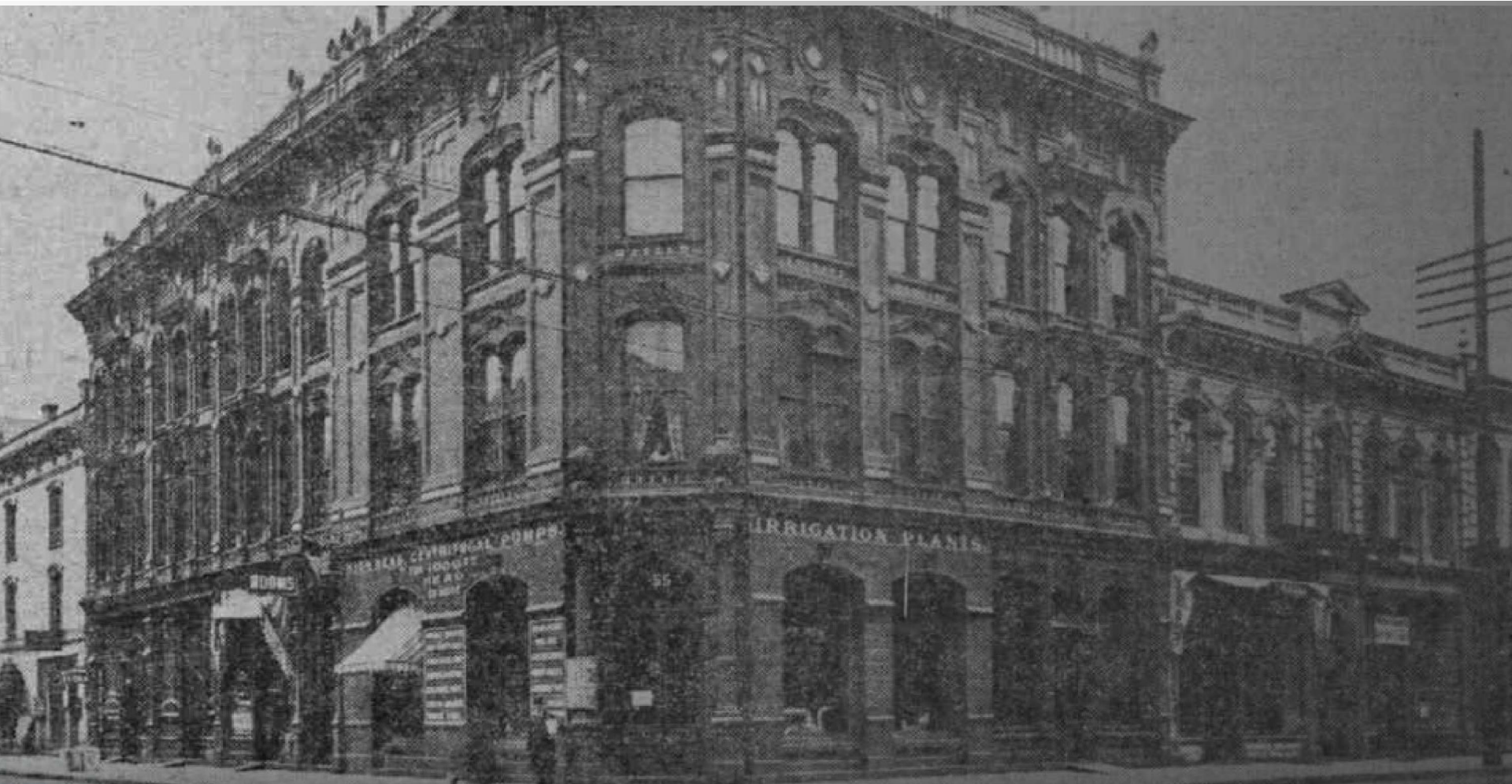
FORMER 1883 REID'S BLOCK BUILDING ON SITE (DEMOLISHED MID 20TH CENTURY)
