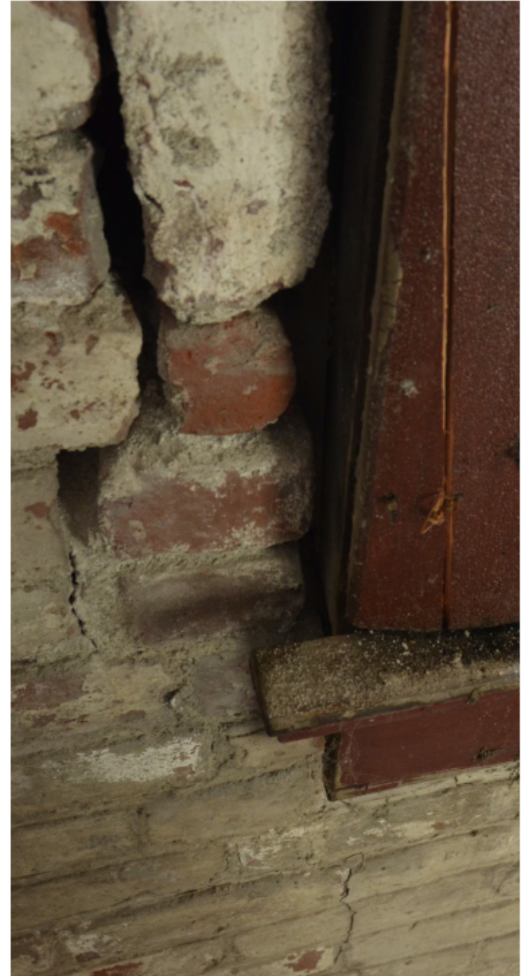
BEFORE: The masonry walls and openings were in extremely poor condition and required full tuck-pointing throughout the interior.
