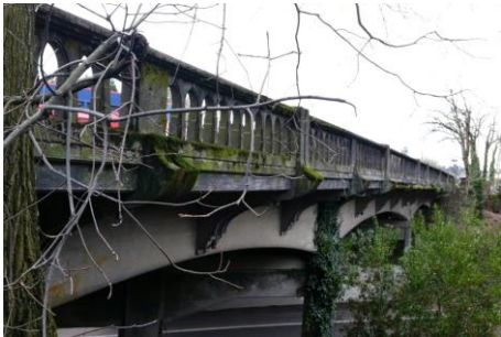
Oregon Electric Railway Overcrossing (replaced)
