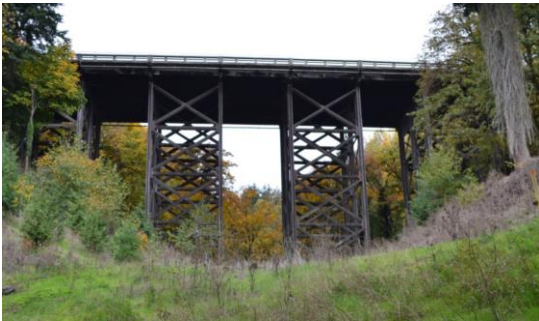
Newbury Viaduct (replaced)
