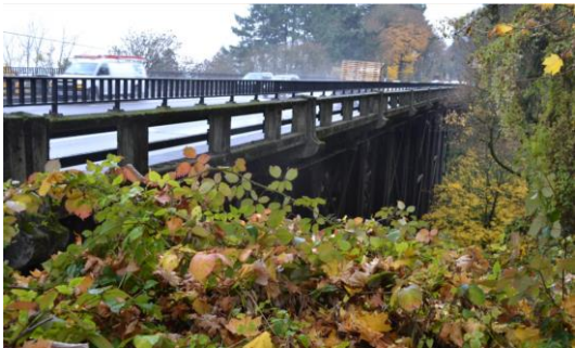
Vermont Viaduct (replaced)
