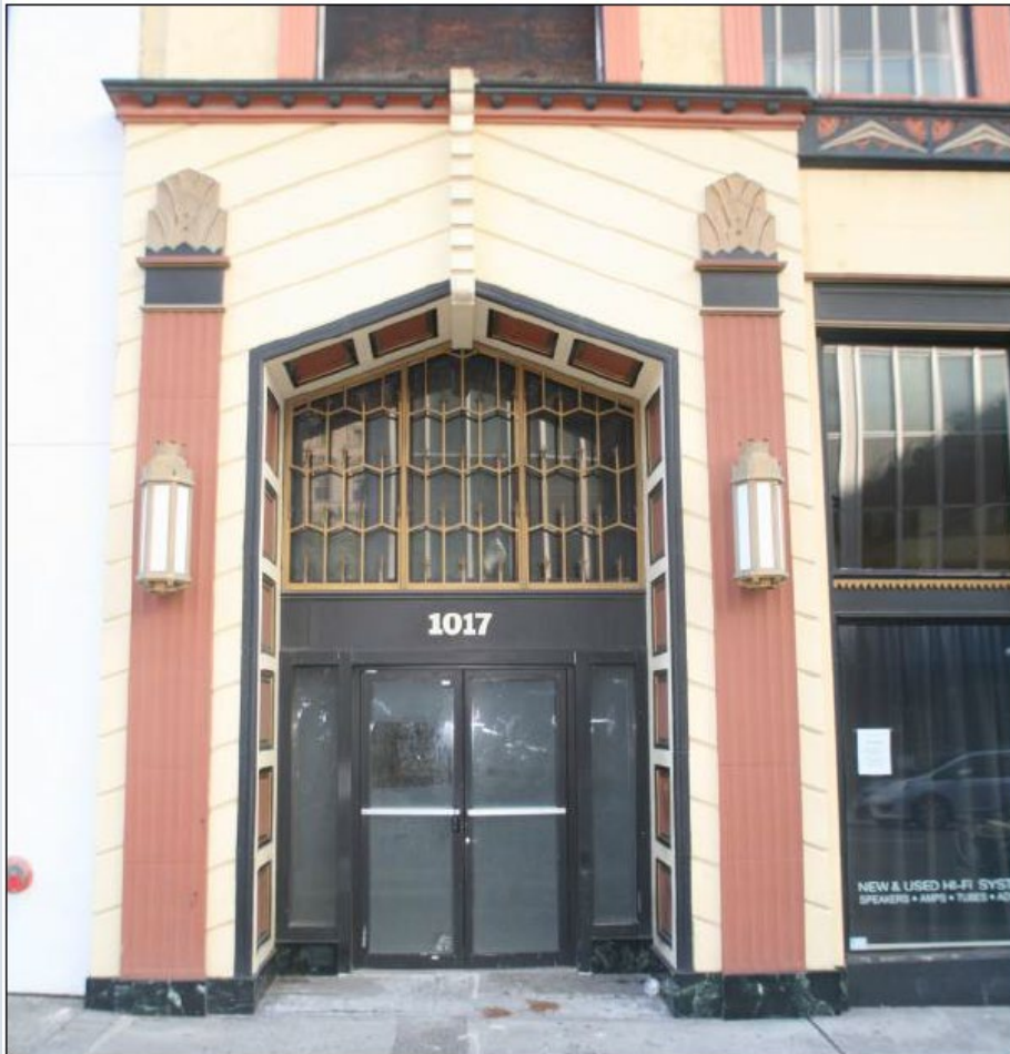
Main Entrance (south elevation)
