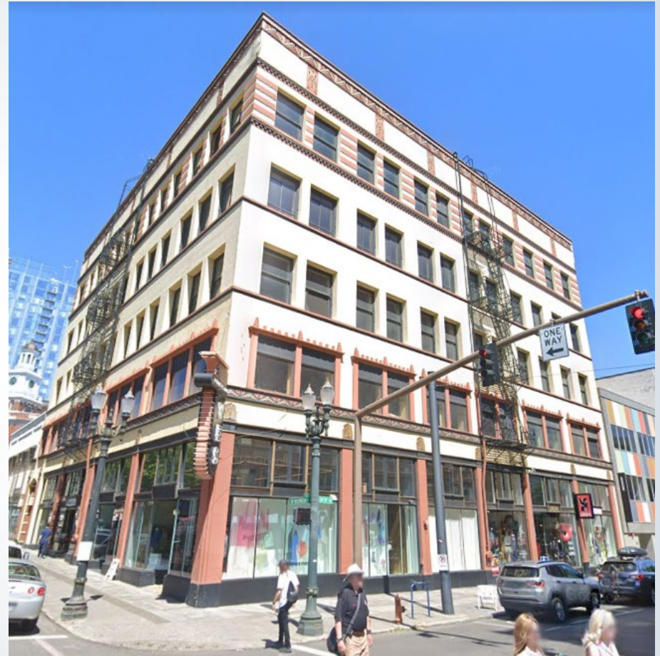
South and east facing façades at corner of SW 10th & Washington
