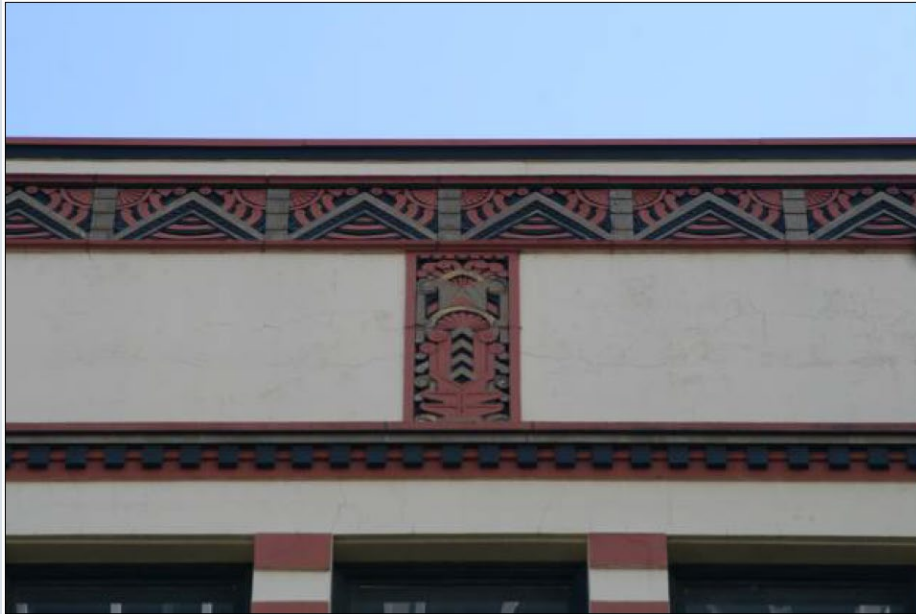
Exterior detail, decorative zig zag cornice
