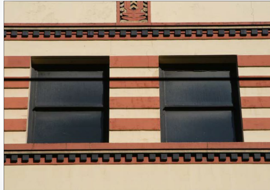
Exterior detail, decorative zig zag trim at fifth floor
