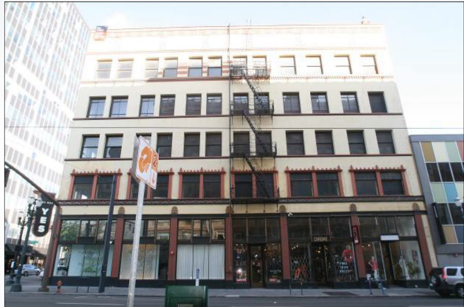
Exterior view, east elevation, looking west from SW 10th Avenue
