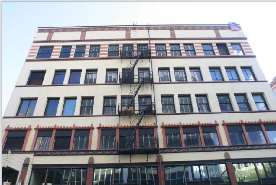
Exterior view, south elevation, looking north from SW Washington Street
