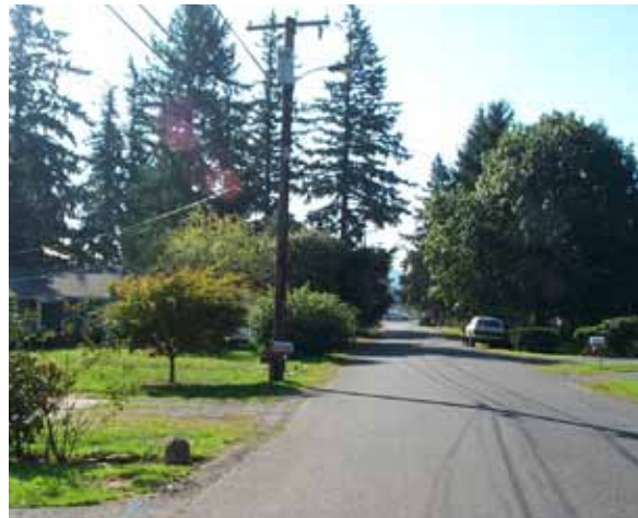
Street in East. Incomplete street; no sidewalks on either side of the street. Are sidewalks necessary, given the relatively low-density development pattern in the area?
