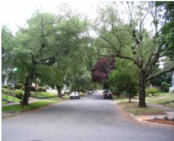
Street in Northeast. Complete street with sidewalks on both sides of the street. A row of on-street parking, street trees and a planter strip buffer pedestrians from traffic.
