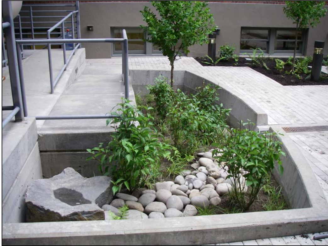
Planters infiltrate or treat stormwater; this planter is monolithically poured concrete in a commercial setting.
