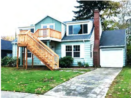
Example of a second-floor entry on the front façade, which would not be allowed
