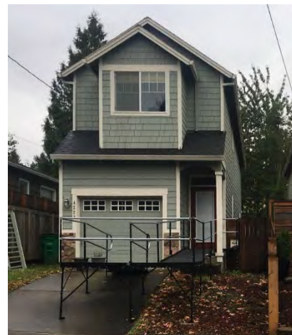
Retrofitting existing development can require extensive and costly modifications.
