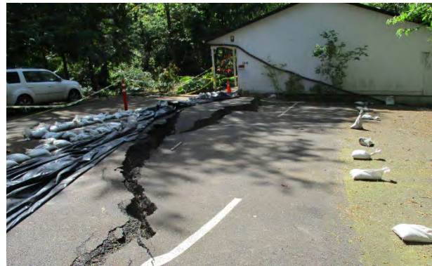
Example of an active deep landslide
