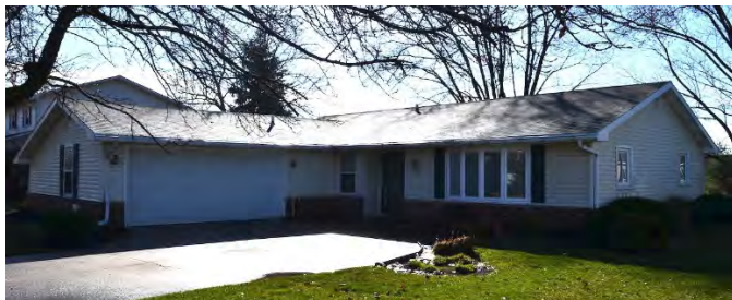
Attached accessory structure
