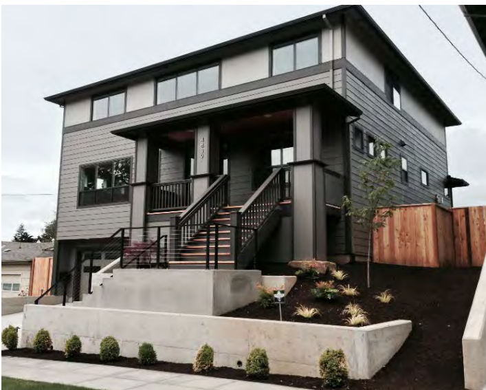
Portland's current code specifies that height measurements be taken from the highest grade next to the house, allowing for potential manipulations of grades to increase a house's height.
