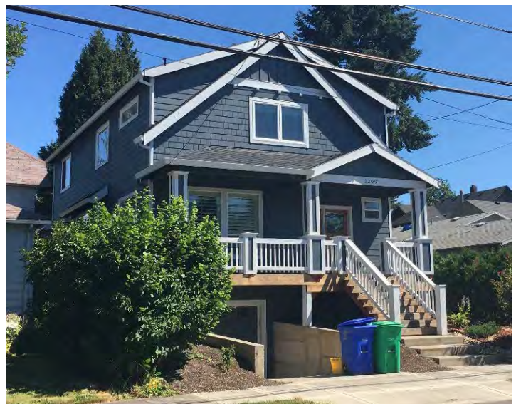
Without limits, dormers (currently not measured when determining a house's height) may begin to look and function like an entire additional story, resulting in a height that is taller than the maximum allowed.
