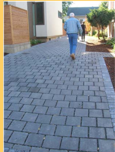
Driveway (above), surfaced with paving blocks, providing shared pedestrian and vehicle access to rear buildings and parking—a space-efficient alternative to requirements for grade-separated walkways (top).
