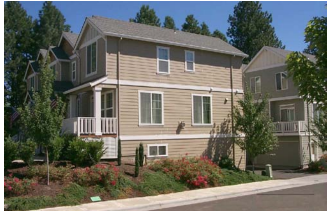
Raised courtyard allows strong relationship to these rowhouse units’ entry porches and living spaces, while lower-level garages are tucked unobtrusively below.
