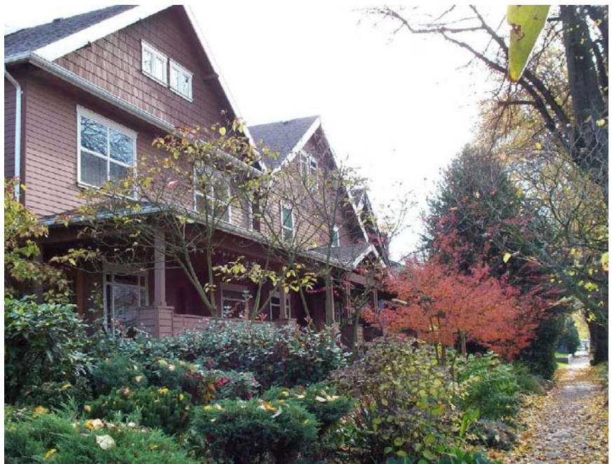
Rowhouses with rear-accessed parking, highlighting how this allows for continuation of the surrounding neighborhood's pattern of landscaped setbacks.
