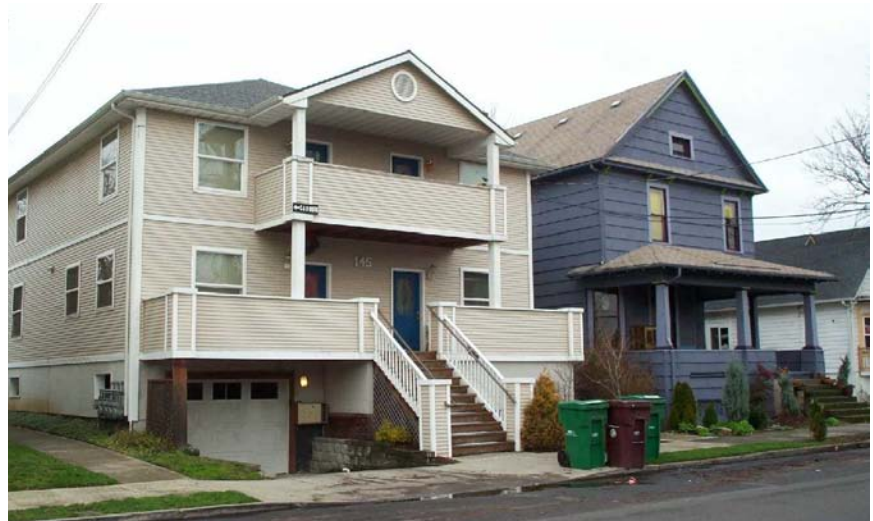
Fourplex with excavated basement parking
