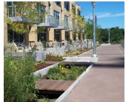
Stormwater planters integrated into the design of shared pedestrian/vehicle space (Meriwether Townhouses)
