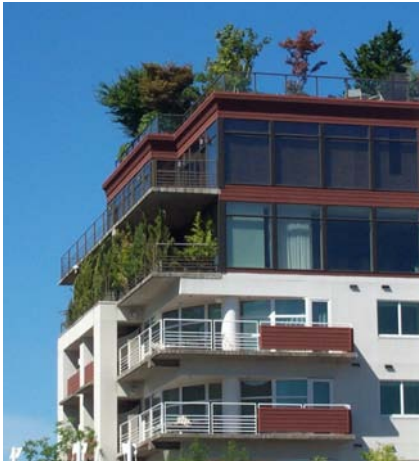
The predominance of glass, combined with the subdued colors, step backs and terrace plantings of upper levels diminish apparent building scale.
