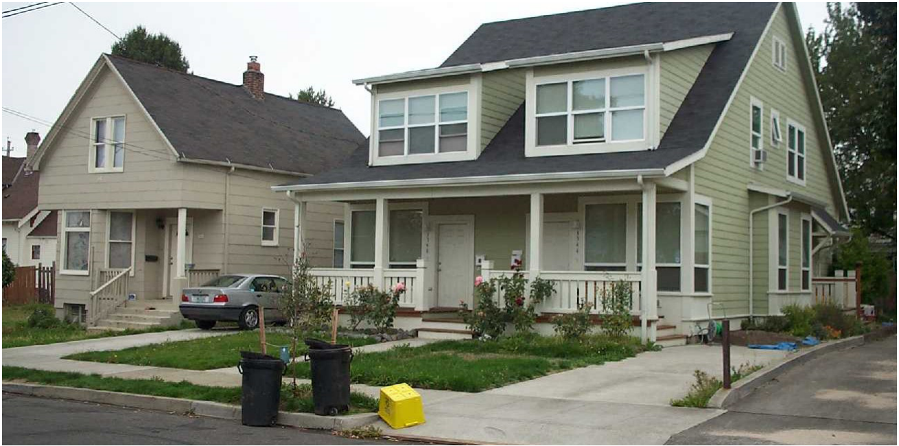
Paired rowhouses with separated parking pads, allowing landscaping to be central. The Office of Transportation generally requires driveways to be paired, but will often allow separated driveways if an on-street parking space is preserved between driveways.
