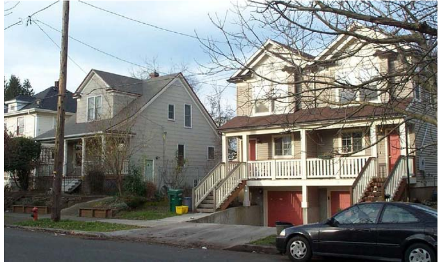
Rowhouses with excavated lower-level garages
