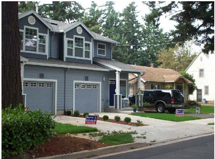
Roof forms set at single-level height help mitigate the scale contrast between these paired rowhouses and the adjacent small cottage.
