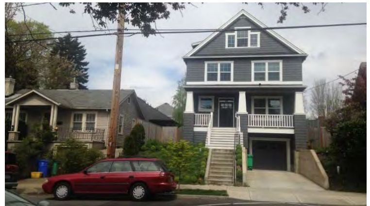
Narrow eaves – common in many new Portland houses – are often the result of current code limits.
