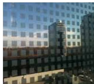
View of fritted window pattern (above) at the OHSU Center for Health and Healing demonstrate how frit patterns can be designed to afford views out (Photo at left is a close-up). Frits can synergistically reduce solar heat gain, afford privacy, and provide visual cues to approaching birds. No collisions have been documented at this building in four seasons of monitoring. Photo: Mary Coolidge
