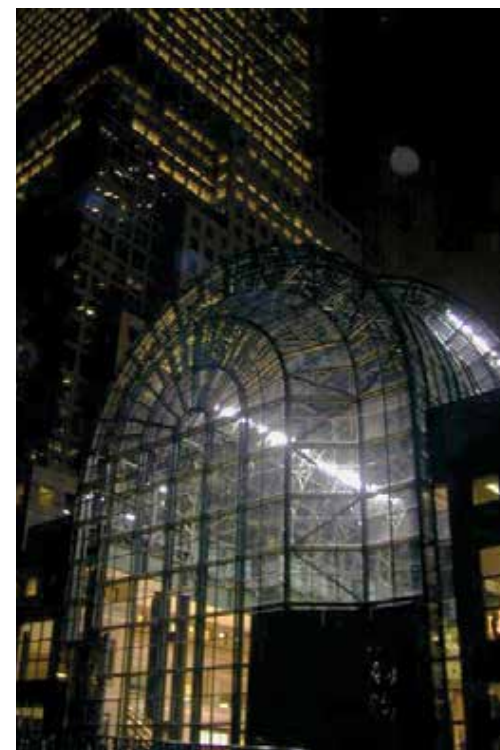
The glass walls of this atrium, coupled with nighttime illumination, create an extreme collision hazard for birds. Photo courtesy of New York City Audubon
