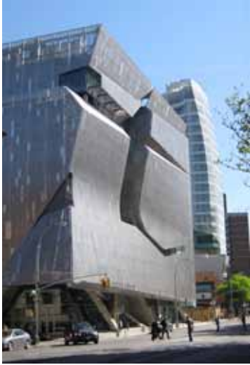
41 Cooper Square in New York City, by Morphosis Architects, features a skin of perforated steel panels fronting a glass/aluminum window wall. The panels reduce heat gain in summer and add insulation in winter while also making the building safer for birds. Photo: Christine Sheppard, ABC
