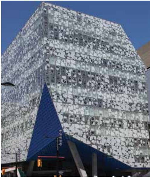
Snohetta's Student Learning Centre at Ryerson University is one of the first constructed under Toronto's design law. Photo by Rick Ligthelm
