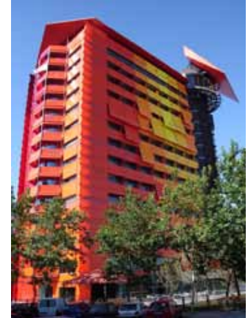
The Hotel Puerta America in Mexico City was designed by Jean Nouvel, and features external shades. This is a flexible strategy for sun control, as well as preventing collisions; shades can be lowered selectively when and where needed. Photo: Ramon Duran
