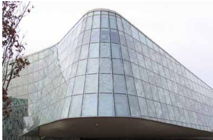
The dramatic City Hall of Alphen aan den Rijn in the Netherlands, designed by Erick van Egeraat Associated Architects, features a façade of etched glass. Photo: Dik Naagtegal
