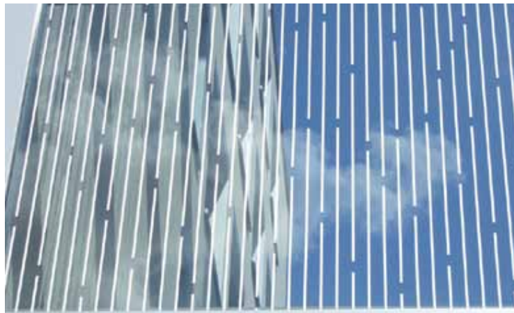
Patterns on the outside of glass, such as that shown above, are more effective than patterns on an inside surface. Photo: Hans Schmid
