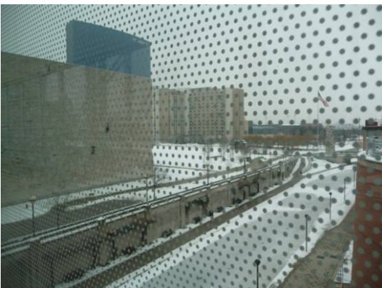
LEFT: This skywalk was intentionally treated with fritting by the Indiana Museum to avoid creating a “feature-related” hazard.
