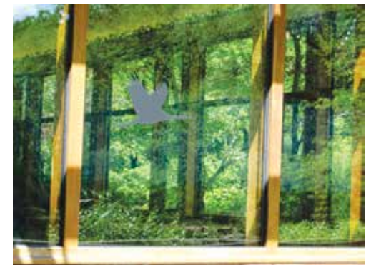
Birds may try to reach vegetation seen through two or more glass walls or windows; the single decal here is not enough to solve the problem, but two or three could do the trick. Photo by Christine Sheppard, ABC
