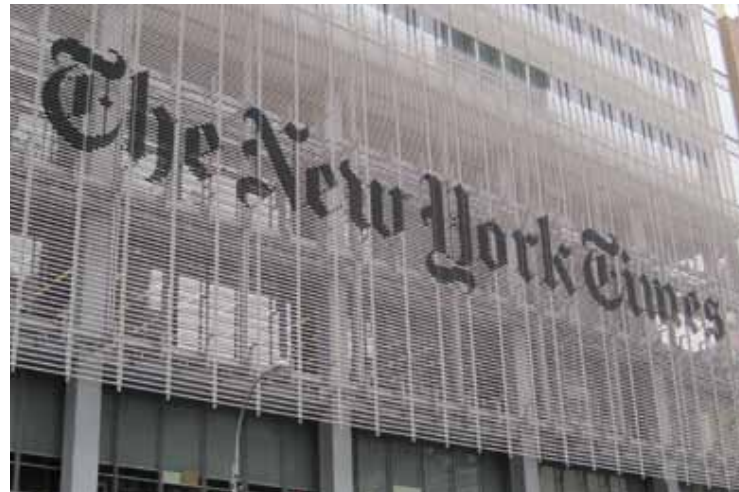
The façade of the New York Times building, by FX Fowle and Renzo Piano, is composed of ceramic rods, spaced to let occupants see out, while minimizing the extent of exposed glass. Photo: Christine Sheppard, ABC
