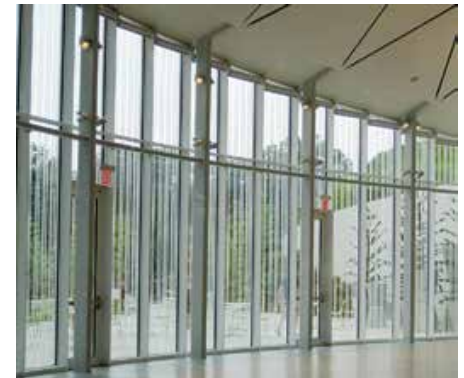
Glass walls and doors at the Brooklyn Botanic Garden's Visitors Center include a custom fritting pattern that meets bird-friendly criteria. Monitoring for collisions after the building opened indicates that the design was successful. Photo by Christine Sheppard, ABC
