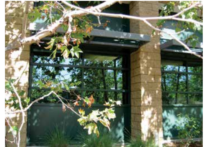
Lower-floor windows are thought to be more dangerous to birds because they are more likely to reflect vegetation. Photo by Christine Sheppard, ABC
