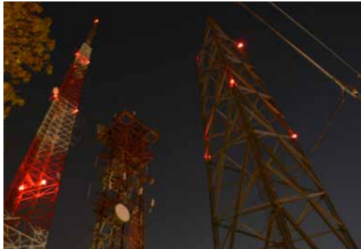
Steady-burning red and white lights are most dangerous to birds. Photo: Mike Parr, ABC
