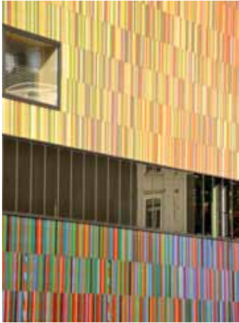
The area of glass on a façade is the strongest predictor of threat to birds. The façade of Sauerbruch Hutton's Brandhorst Museum in Munich is a brilliant example of the creative use of non-glass materials. Photo: Tony Brady
