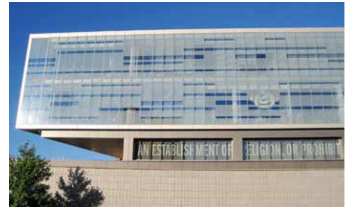
Newhouse III, designed by Polshek Partnership Architects, is part of Syracuse University's S.I. Newhouse School of Public Communications. This building incorporates an undulating, fritted glass façade with the words of the first amendment etched in letters six feet high along the base. Photo by Christine Sheppard, ABC
