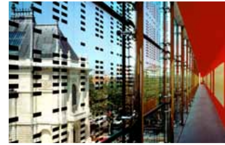
External frit, as seen here on the Lile Museum of Fine Arts, by Ibos and Vitart, is more effective at breaking up reflections than patterns on the inside of the glass. Photo: G. Fessy
