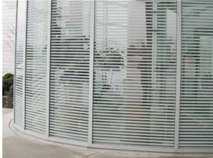
Dense stripes of internal frit on University Hospital's Twinsburg Health Center in Cleveland, by Westlake, Reed, Leskosky will overcome virtually all reflections. Photo: Christine Sheppard, ABC
