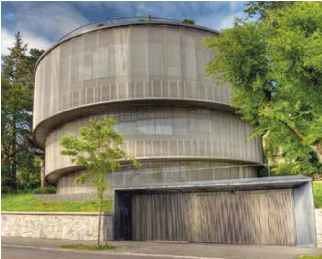
The steel mesh enveloping Zurich's Cocoon in Switzerland, designed by Camenzind Evolution, Ltd, provides privacy, reduces heating and cooling costs, and protects birds, but still permits occupants to see out. Photo by Anton Volgger
