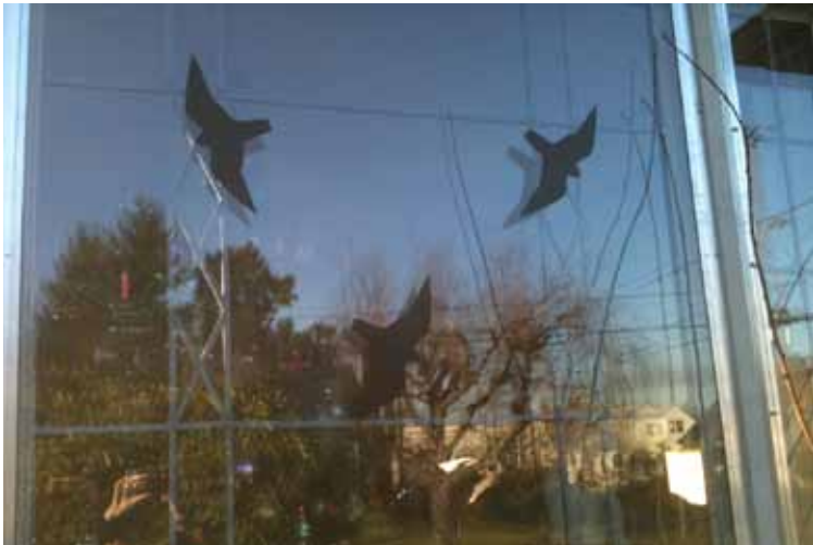
Silhouettes placed every 12 inches on the exterior of this residential window are spaced too far apart to reliably eliminate all strikes, but will likely reduce strike incidence.
