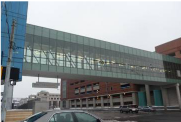
LEFT: A transparent glass skywalk poses a “feature-related” hazard.
