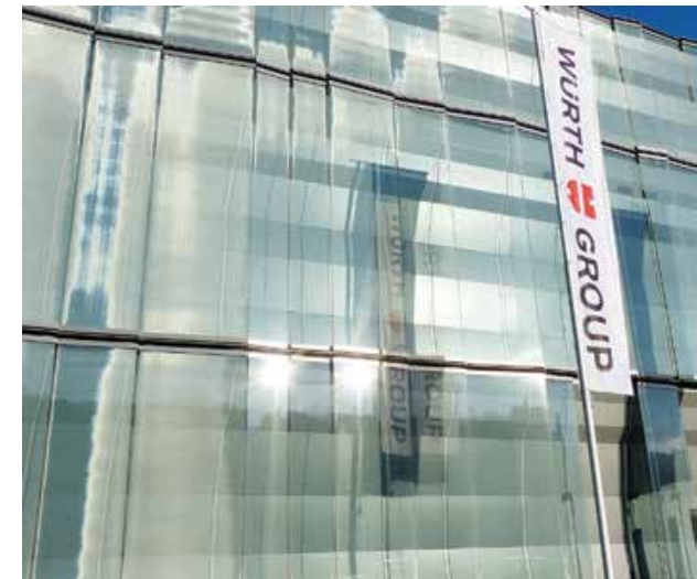
The façade of the WÜRTH Building in Switzerland is mostly glass, laminated with a fabric that is black on the inside but aluminium-coated outside. The inner surface delivers good visibility, and the fabric provides shade and interesting visual effects outside. Preliminary studies by the Swiss Ornithological Institute suggest that the materials used in this building may also deter bird collisions. Photo by Hans Schmid
