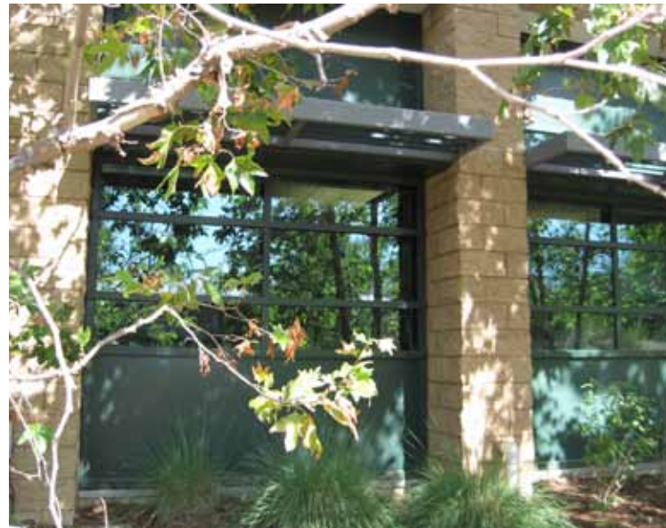
Lower floor windows are thought to be more dangerous to birds because they are more likely to reflect vegetation. Photo: Christine Sheppard, ABC
