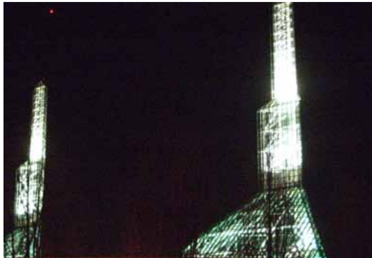
The iconic spires of the Oregon Convention Center feature unshielded light fixtures, rendering the spires visible for miles; though controversial, dimming or extinguishing these lights during migration season could reduce a potential collision hazard. Photo: Mary Coolidge
