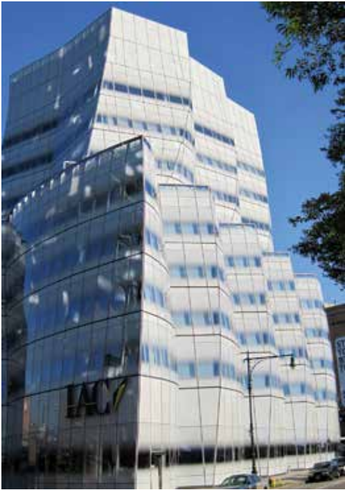
While some internal fritted glass patterns can be overcome by reflections, Frank Gehry's IAC headquarters in Manhattan is so dense that the glass appears opaque. Photo by Christine Sheppard, ABC
