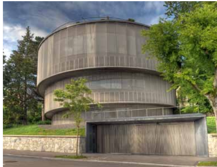
The steel mesh enveloping Zurich's Cocoon in Switzerland, designed by Camenzind Evolution Ltd, provides privacy and protects birds, but still permits occupants to see out. Photo: Anton Volgger
