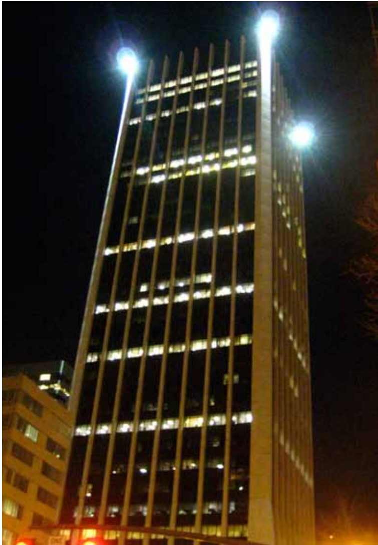
The height of the Wells Fargo Tower, coupled with its corner floodlights, make this building a potential collision hazard for migrants. Dimming or extinguishing exterior and rooftop lighting during migration season can help reduce collision hazards. Photo: Mary Coolidge
