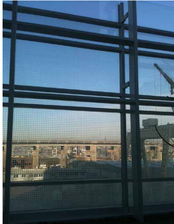
View of fritted window pattern (above) at the OHSU Center for Health and Healing demonstrate how frit patterns can be designed to afford views out (Photo at left is a close-up). Frits can synergistically reduce solar heat gain, afford privacy, and provide visual cues to approaching birds. No collisions have been documented at this building in four seasons of monitoring. Photo: Mary Coolidge
