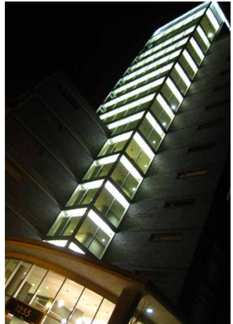
Light spill is apparent from this stairwell in the Pearl District, and could be minimized by exterior shielding. Photo: Mary Coolidge
