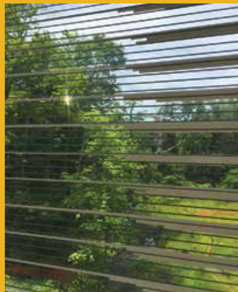
Glass detail, showing frit pattern
