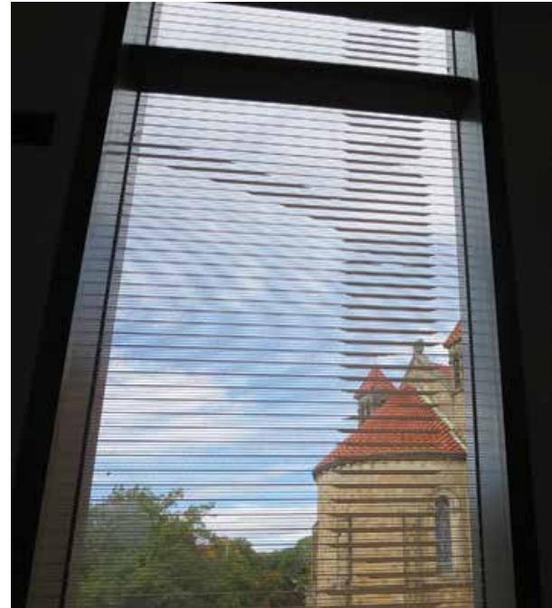
A custom frit pattern was designed by Ennead Architects for Vassar College’s Bridge for Laboratory Sciences building. Elements of the pattern occur on two separate surfaces, increasing visibility to birds in flight, who will see a constantly changing pattern that may appear to move. Photo by Christine Sheppard, ABC
