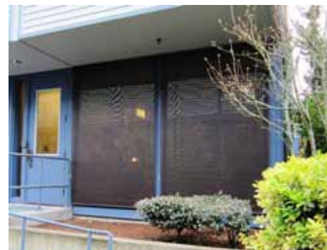
Six reflective windows on the Port of Vancouver administrative building are slated for a pilot installation of roll-up solar shades, which will serve the dual purpose of softening incoming light and reducing strike hazards. Top photo shows window with shades up and bottom shows the window with the shades down. Photo PoV.
