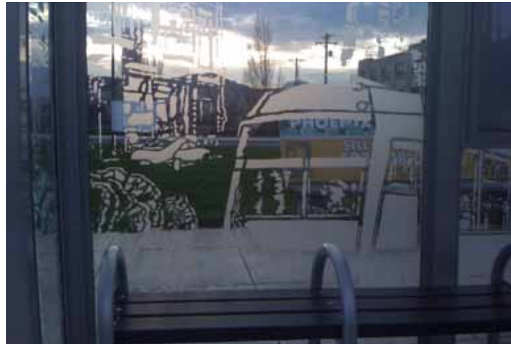
Designwork on TriMet bus shelters has been shown to help to reduce vandalism and also marks the freestanding glass for birds. Photo: Mary Coolidge
