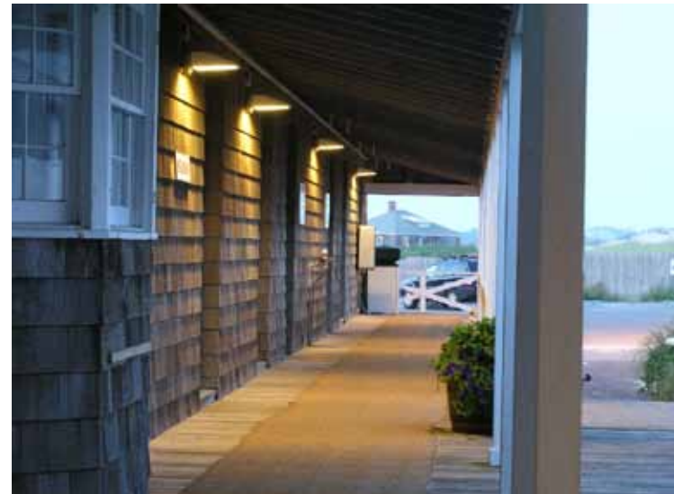
Shielded lights, such as those shown above, cut down on light pollution and are much safer for birds. Photo: Susan Harder
