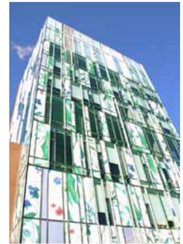
Issues of cost prompted Hariri Pontarini Architects, in a joint venture with Robbie/Young + Wright Architects, to revise a planned glass and limestone façade on the School of Pharmacy building at the University of Waterloo, Canada. The new design incorporates watercolors of medicinal plants as photo murals. Photo: Anne H. Cheung
