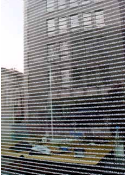
The glass facade of SUVA Haus in Basel, Switzerland, renovated by Herzog and de Meuron, is screen-printed on the outside with the name of the building owner. Photo: Miguel Marqués Ferrer
