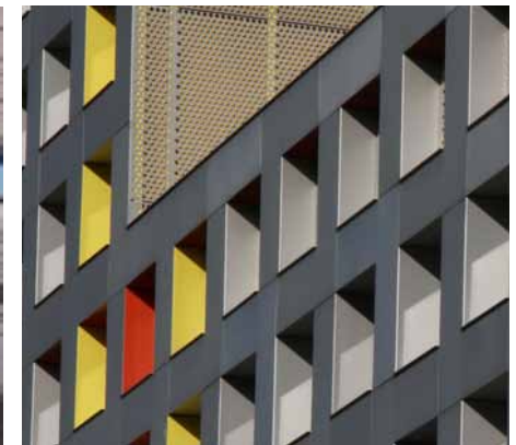
Deeply recessed windows, such as these on Stephen Holl's Simmons Hall at MIT, can block viewing of glass from oblique angles. Photo: Dan Hill
