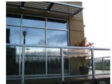
Transparent handrails are a dangerous trend for birds, especially when they are in front of vegetation. Photo: Mary Coolidge
