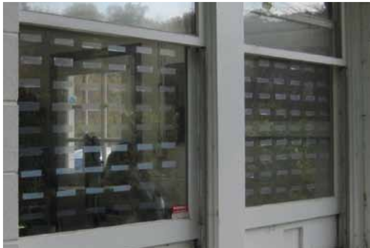
Tape decals (Window Alert shown here) placed following the 2 x 4 rule can be effective at deterring collisions. Photo: Christine Sheppard, ABC
