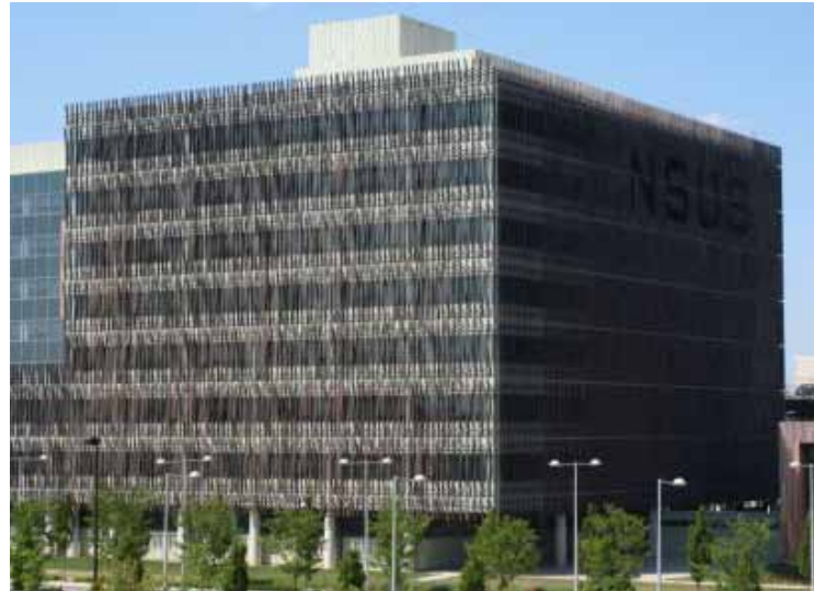
The U.S. Census Complex in Suitland, Maryland, designed by Skidmore, Owings, Merrill, features a brise soleil that shades the curtain wall. Wavy vertical fins of marine-grade, white oak reduce sun glare while eliminating glass reflections. Photo: Esther Langan
