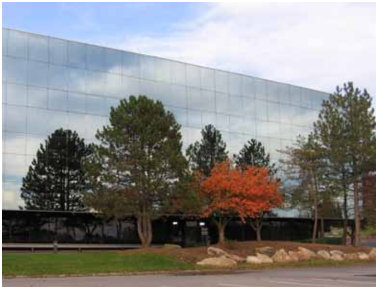
The mirrored glass of this office building reflects nature so perfectly that it is easy to see how birds mistake reflection for reality. Photo: Christine Sheppard, ABC
