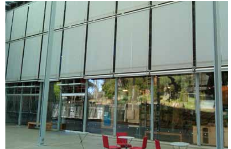
External shades on Renzo Piano's California Academy of Sciences in San Francisco are lowered during migration seasons to eliminate collisions. Photo: Mo Flannery
