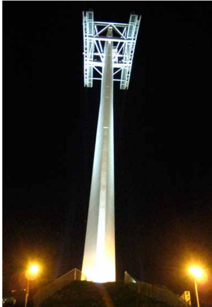
Unshielded, upward-directed floodlights at the base of the OHSU Tram Tower contribute directly to Portland's skyglow; existing fixtures which light the tram from above could instead be utilized as the primary lighting system. Photo: Mary Coolidge
