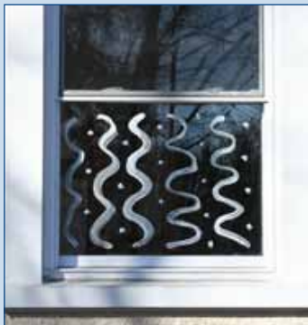
Tempera paint is a washable, long-lasting, and non-toxic solution to preventing bird/window collisions. Photo: Christine Sheppard, ABC.
