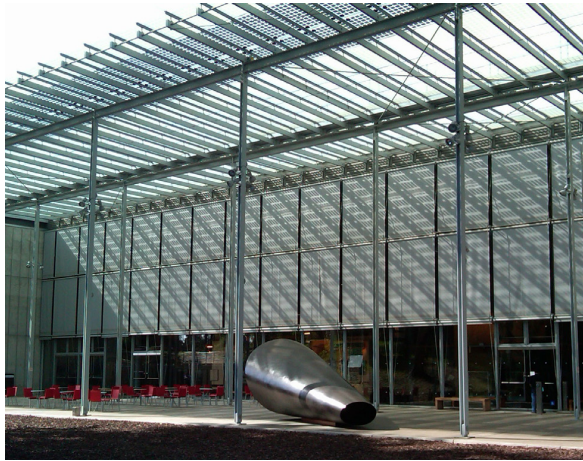
ABOVE: The California Academy of Sciences uses external screens 24 hours per day during spring and fall migration to reduce bird/building collisions.
