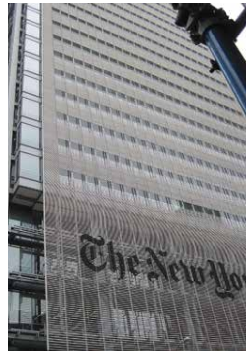
The façade of the New York Times building, by FXFOWLE and Renzo Piano, is composed of ceramic rods, spaced to let occupants see out while minimizing the extent of exposed glass—good for controlling heat and light, and safe for birds. Photo by Christine Sheppard, ABC
