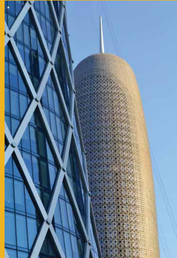
The Burj Qatar, designed by Jean Nouvel, was named Best Tall Building Worldwide in 2012. The façade, created with multi-layered screens, expresses local culture while providing protection from high temperatures and sand. Photo by Marc Desbordes
