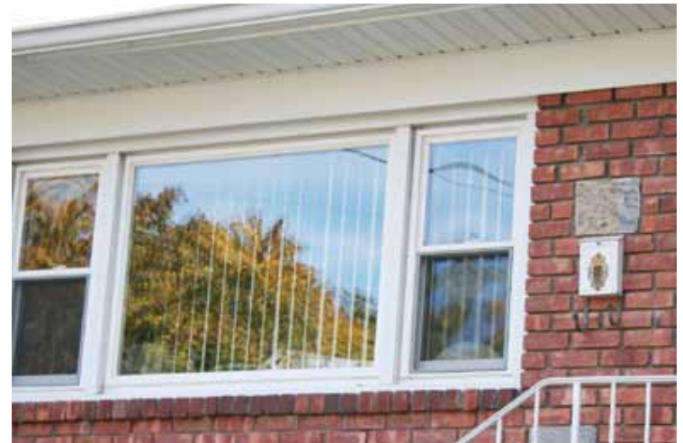
Reflections on home windows are a significant source of bird mortality. Partially opened vertical blinds may break up reflections enough to reduce the hazard to birds. Photo: Christine Sheppard, ABC
