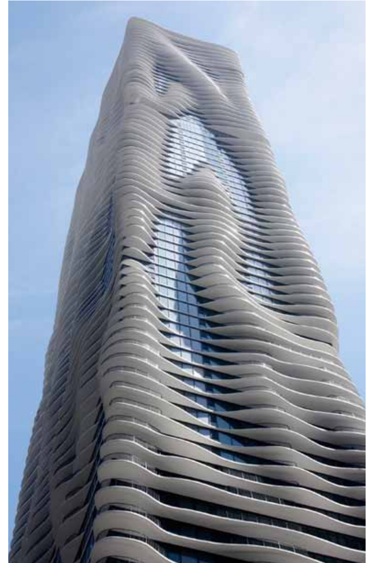
The Studio Gang's Aqua Tower in Chicago was designed with birds in mind. Strategies include fritted glass and balcony balustrades. Photo: Tim Bloomquist
