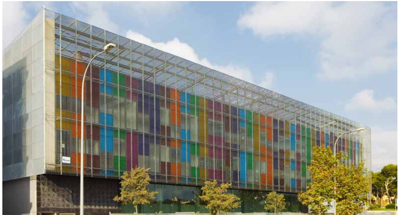
Boris Pena's Public Health Office building in Mallorca, Spain, sports a galvanized, electro-fused steel façade which deflects bird strikes. Photo: Boris Pena
