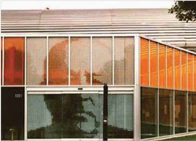
The IIT Student Center in Chicago uses faceted glass, Panelite panels and a dot matrix pattern (above) in its facade. These elements create visual noise which is perceptible to birds.
