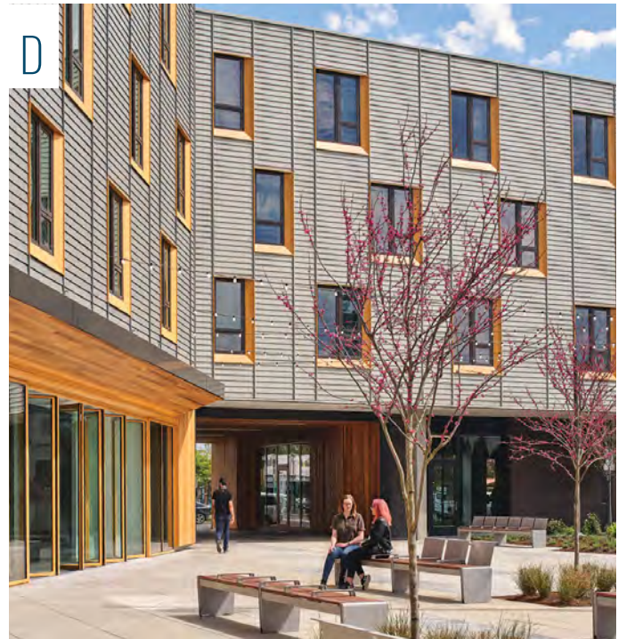
SAME SPACE - DIFFERENT PHOTO: credit: HOLST ARCHITECTURE Expressing building function and hierarchy by emphasizing the ground floor with high quality materials and using repetition in the design and placement of upper level openings and materials.
