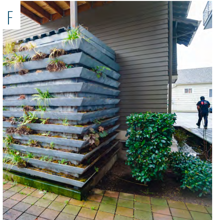
GARBAGE BEHIND BUILDING AND ARTFULLY SCREENED WITH PLANTER
