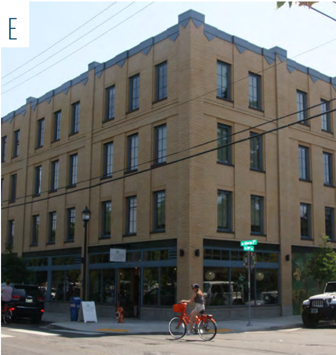
Evoking early streetcar architecture forms and patterns within Inner Neighborhood Centers and along Neighborhood Corridors. Alberta, NE Alberta and NE 19th
