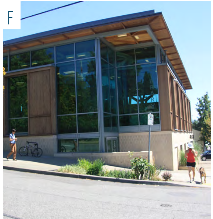
Designing buildings that integrate topography while maintaining high ground floor window visibility. This building optimizes a retaining wall to support sitting and pausing within Western Neighborhood centers. Hillsdale, SW Sunset Blvd and SW Dewitt
