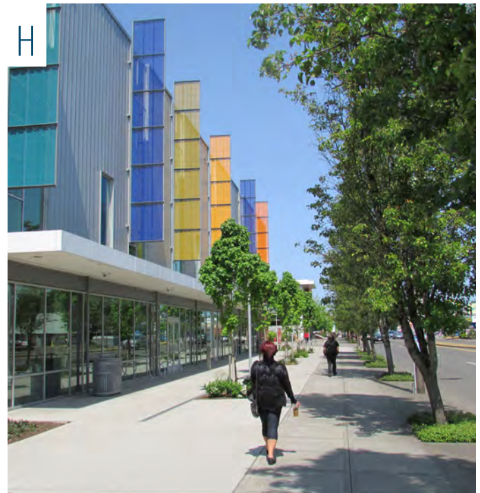
Transforming Civic Corridors into green, lush pedestrian-oriented streetscapes. This frontage sets back and devotes space for a double alley of trees to encourage walking on a busy street. Jade District, SE 82nd and SE Division
