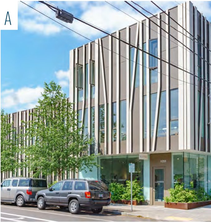
Applying materials and forms consistently. This building undulates through both the pattern of its façade and on the ground floor, where entries are tucked in and planters push out toward the sidewalk. Northwest District, NW 19th and NW Overton
