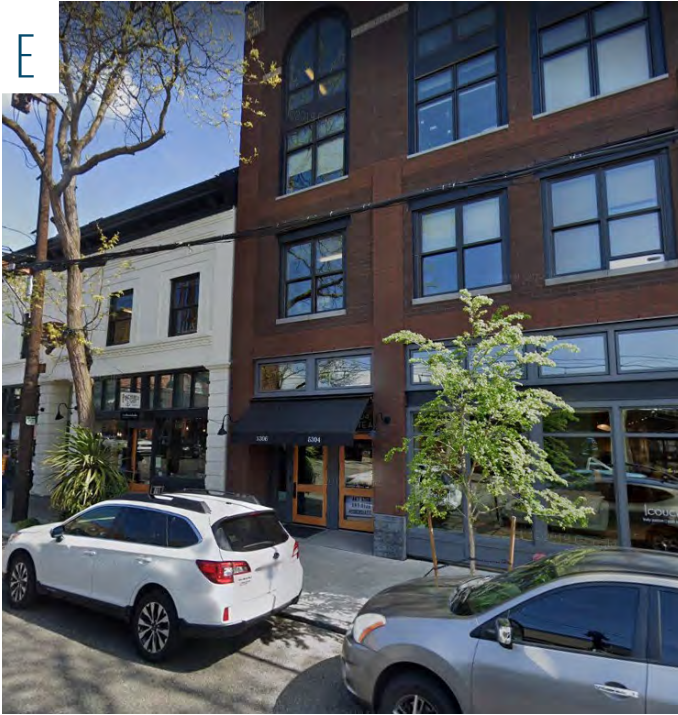
ALIGNING BELT COURSES AND WINDOW HEIGHTS. NOTE: THIS IS A SCREEN SHOT
