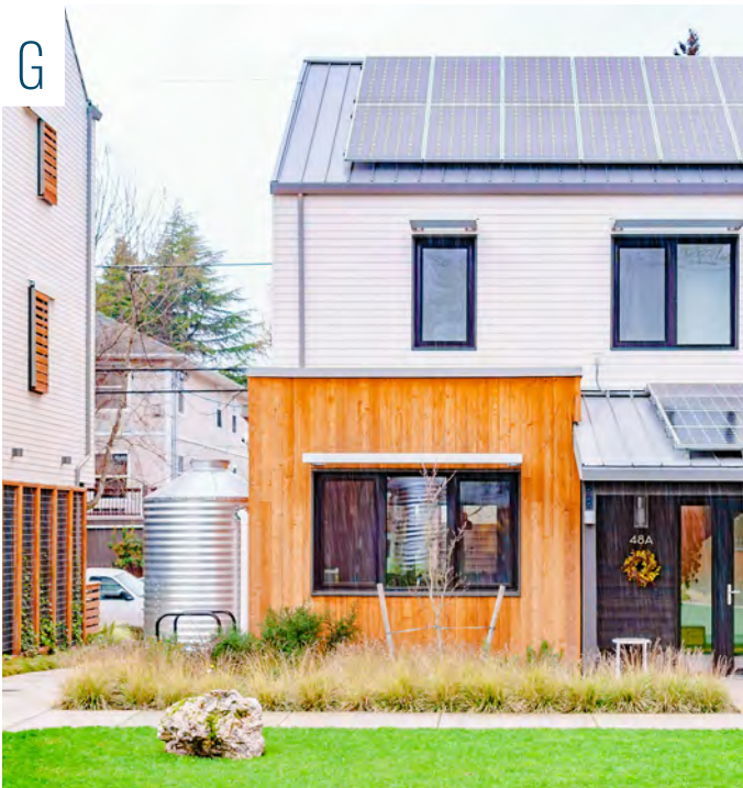
SAME SPACE - DIFFERENT PHOTO: Striving towards net zero with features that include photovoltaic panels on all south-facing roofs, triple-paned windows to limit the amount of hot and cold air and cisterns for collecting rainwater.
