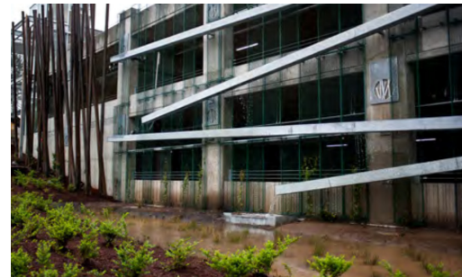
Stormwater improvements along the MAX Orange Line.
