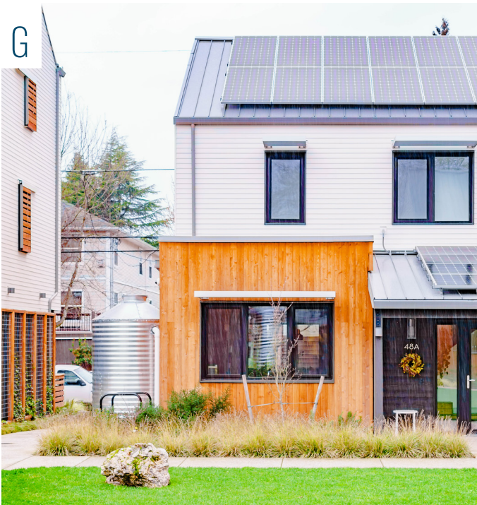
SAME SPACE - DIFFERENT PHOTO: Striving towards net zero with features that include photovoltaic panels on all south-facing roofs, triple-paned windows to limit the amount of hot and cold air and cisterns for collecting rainwater. Eliot, NE Williams and NE Tillamook SEPTEMBER 2019
