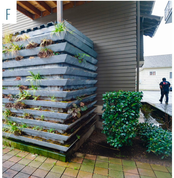
GARBAGE BEHIND BUILDING AND ARTFULLY SCREENED WITH PLANTER
