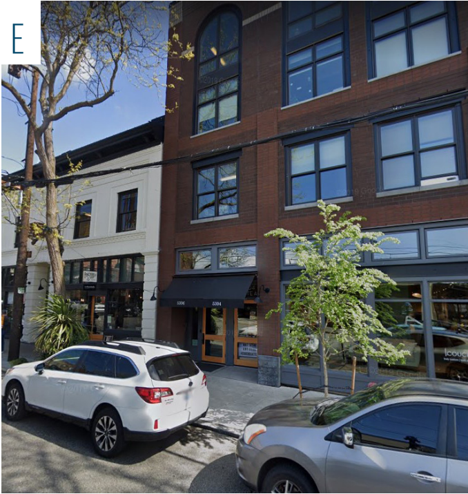
E ALIGNING BELT COURSES AND WINDOW HEIGHTS. NOTE: THIS IS A SCREEN SHOT
