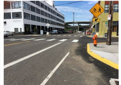
Before and after: A crossing improvement at SE Water and Taylor, funded by Fixing Our Streets.
