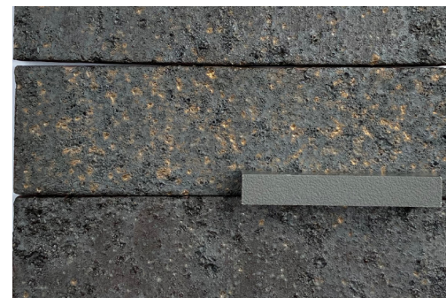
2 Dark Colored Brick & Matching Mortar
