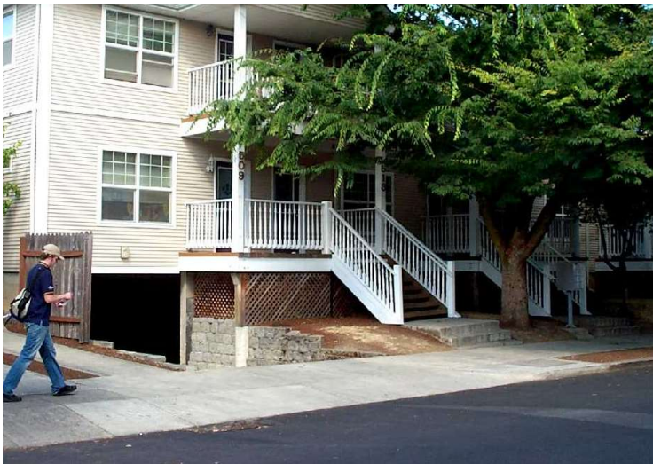
Driveway ramp providing access to below-grade structured parking. Amendments to the Measuring Height section will allow for building height to be measured from the sidewalk elevation, instead of being based on the low point of the driveway ramp.
