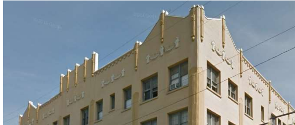
Historic example of parapets providing roofline variety.
