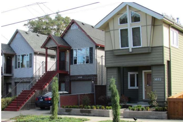
House (center) with long run of stairs that would not meet the distance from grade standard.
