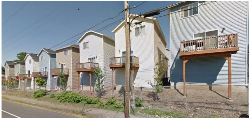
Multi-dwelling zone development (multiple detached houses) with no pedestrian connections to the adjacent transit street. Proposed amendments to pedestrian standards in conjunction with main entrance requirements would prevent this lack of orientation to the street.
