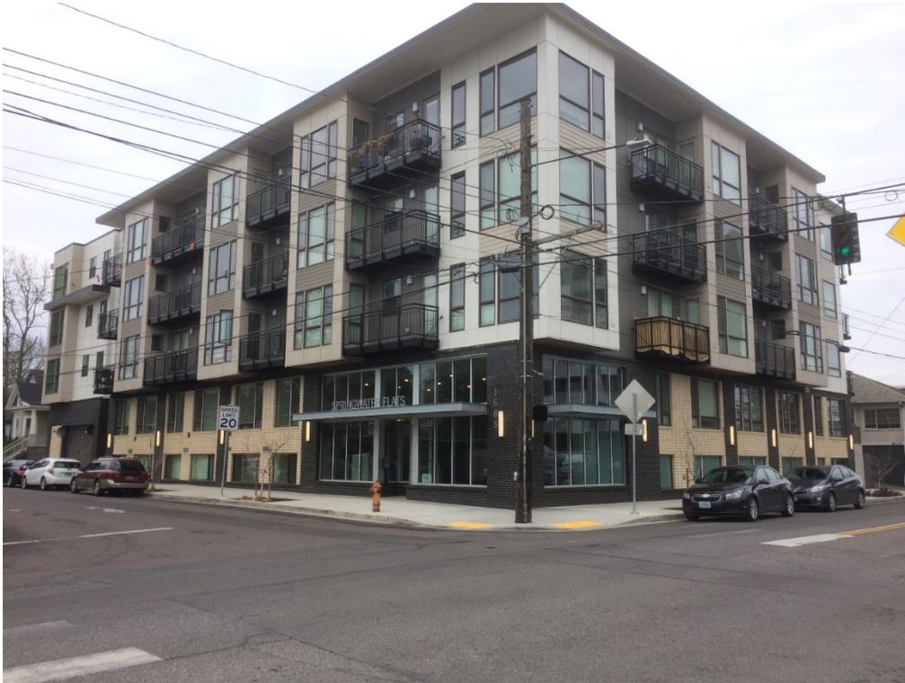
Photo 2a (east side) and 2b (north front and west side). Morgan building, SE Tacoma and 17<sup>th</sup>. Visible rooftop structures on the side of a building increase building mass (QR21). On the sides at the property line color and texture are used to avoid a blank wall (proposed new Public Realm standard). The building advertises that there is an ecoroof, which is not visible to the public (QR22).
