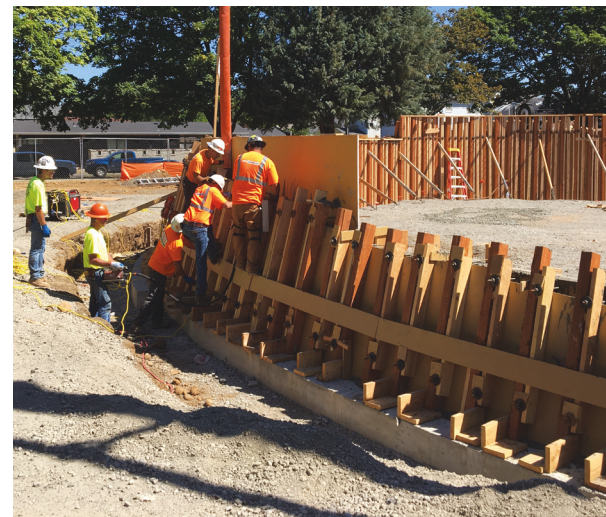
Glenhaven Park Playground construction
