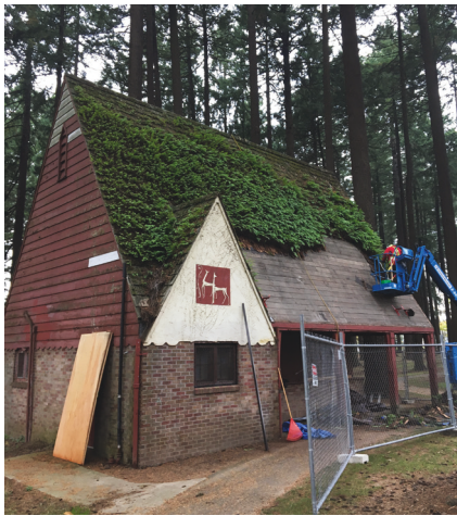
Sellwood Park Kitchen Roof construction
