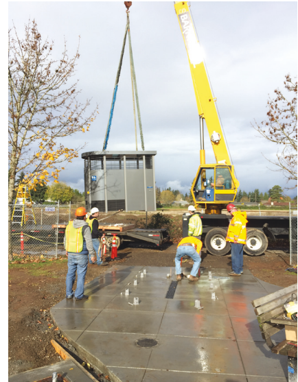
Raymond Park Loo construction
