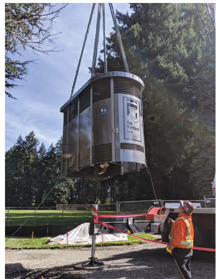
Pier Park construction
