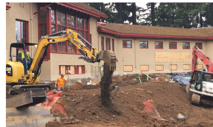
Peninsula Pool construction
