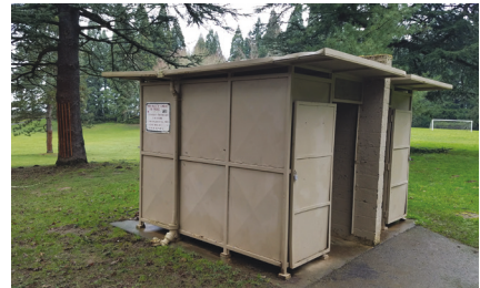
Pier Park restroom (before)
