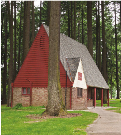
Sellwood Park Kitchen Roof (after)
