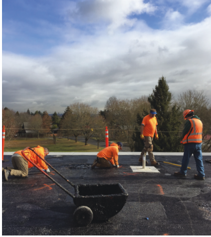
St. Johns Community Center roof construction
