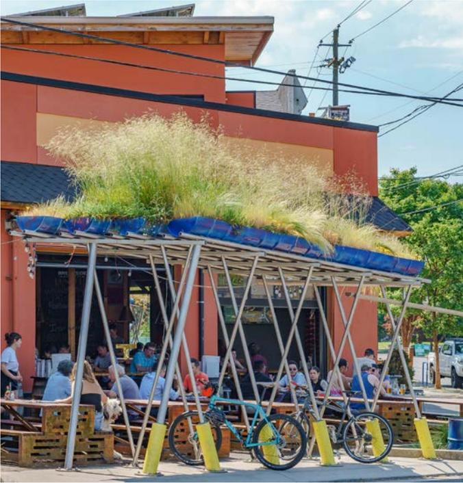
Designing stormwater runoff systems to be multi-functional. This installation manages stormwater, covers bicycle parking, and serves as public art.
