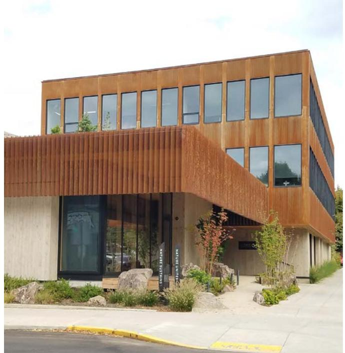
Sourcing regionally harvested and locally manufactured materials, including Cross-Laminated Timber (CLT), weathering steel, Oregon juniper, cedar, and river rock and boulders.
