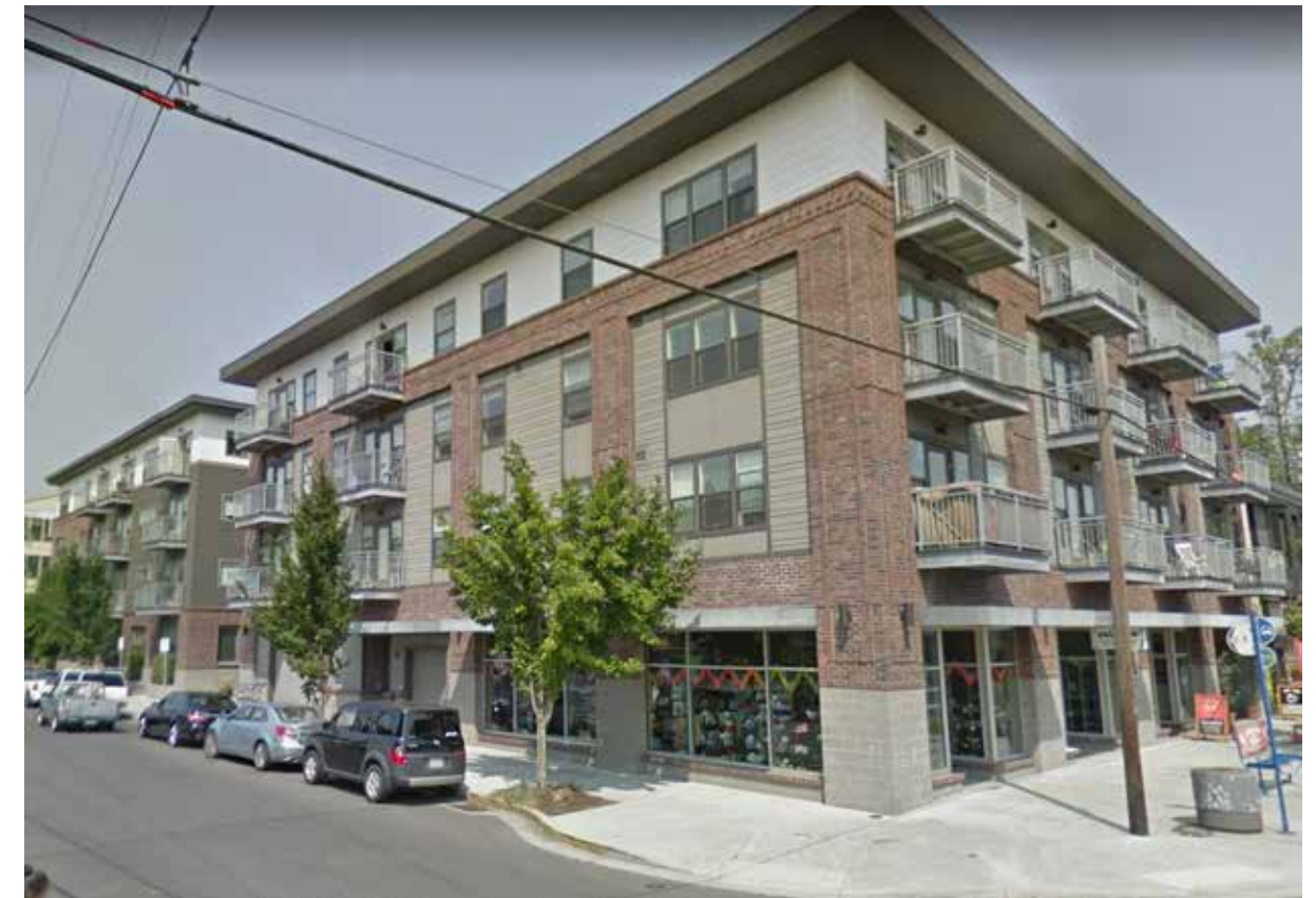
STREET VIEW CORNER SE DIVISION X SE 37TH AVE
